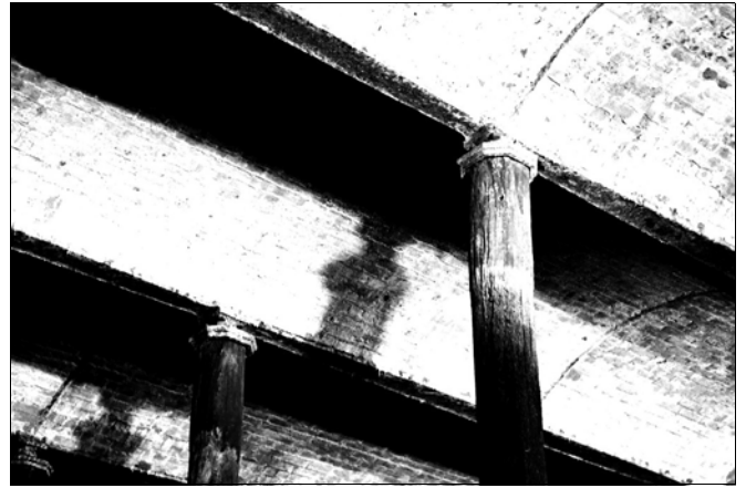
Detail of the interior of the Crown St Reservoir roof, showing an ironbark column, cast-iron column capitals and brick jack arches supported by the cast-iron girders. The dark lines following the curve of the jack arches are the underside of the cast-iron cross stays. Photo C. Doring, 1991.
