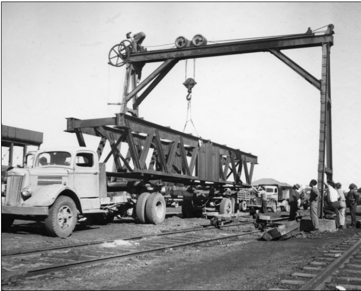
Unloading the jinker using the goods yard gantry crane at Kempsey railway station.
