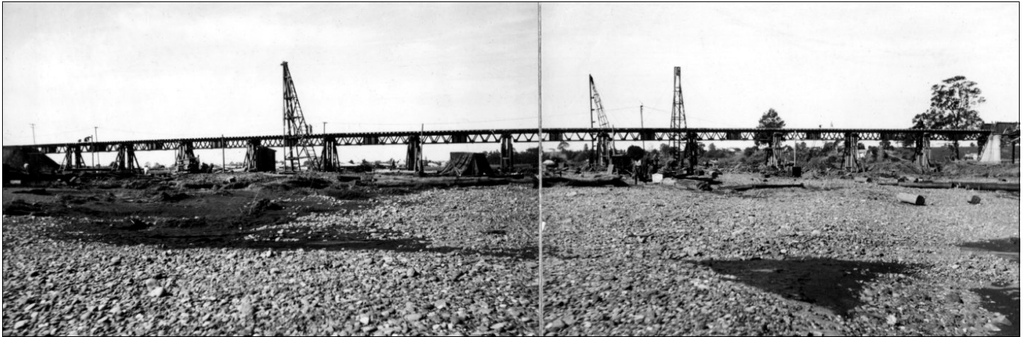
The completed 'temporary' viaduct. It remained in use for 16 years. The view is from the west - the same as the panoramic view of the wrecked viaduct on the third page of this story. The end of the plate web girder at the south end of the viaduct can just be seen on the right. Source: NSW Photo ARHS 126899.
