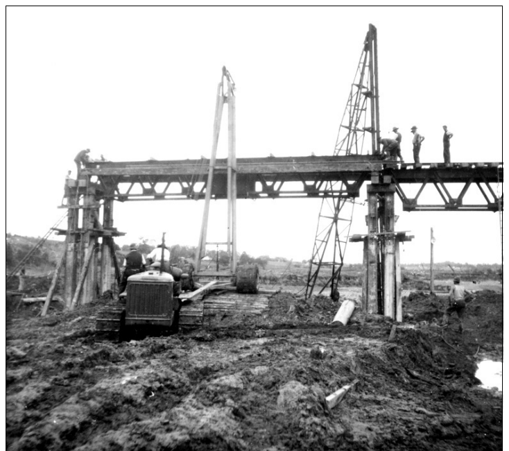
Image above: A wrought iron Warren truss has been rolled forward on falsework and lifted by the caterpillar crane. The NSW caption for this photo draws attention to the mud which persisted for the duration of the job.
