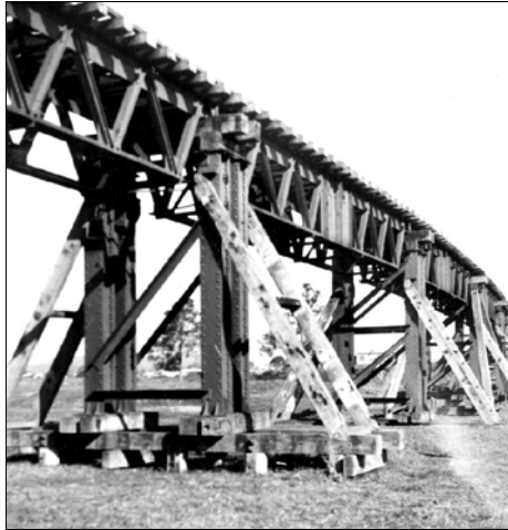
Image Upper Right: The thirteen truss spans were parked on the undamaged No.3 viaduct until the new piers were ready to receive them. Source: NSW Photo ARHS 126886.
