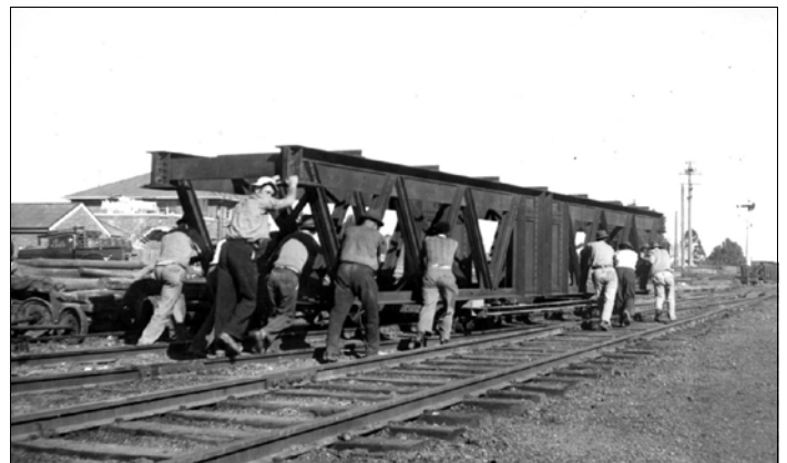
Image Right: Muscle power was used to propel the seven-plus ton assembly for half a mile to its place of use.
