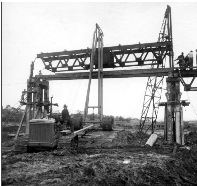
Image above: A wrought iron Warren truss has been rolled forward on falsework and lifted by the caterpillar crane. The NSW caption for this photo draws attention to the mud which persisted for the duration of the job.
