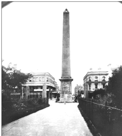
Ventilation Shaft, Erected A.D. 1857 George Thornton Mayor, City of Sydney. City of Sydney File 067/067207, A268.
