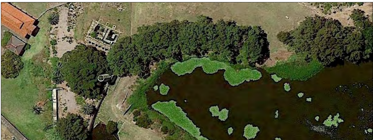
Not the least of the survivals are the archaeological ruins of one of Bell's major works – the Botany Water Pumping Station. On the left in this Google Earth image from 2018, we see the tiled roof of the much later Botany Sewage Pumping Station. Just to its right (east) we see the excavated operating floor level of the Engine House. It was exposed and the pump pits cleaned out in 1995. Along the outside of the north wall are the 3 base plates of the 3 pressure vessels. Due south of the Engine House are the remains of the tall chimney (partly demolished as a danger to aircraft). To the left of the chimney, the Boiler House is hidden under a big fig tree. The Engine Pond is to right of the chimney. – Ed.
