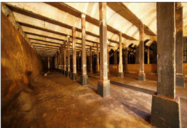
Image at Left: The interior of the reservoir photographed in 2009. Shows ironbark columns, upside down fish-belly girders and brick jack arches.
