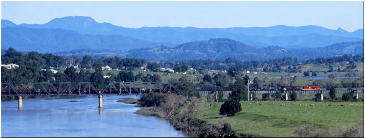
The Kempsey Bridge viewed from the East (downstream) and showing most of the original steel spans over the River (left) and part of a 1960s viaduct over the Flood Plain (right). A long goods train is crossing the bridge and heading for Queensland. No photograph showing the complete crossing with the original timber trestle viaduct, could be found.. Photographer Neil Munro, 31 st May 1983. Source: NSW Photo ARHS 451909.
