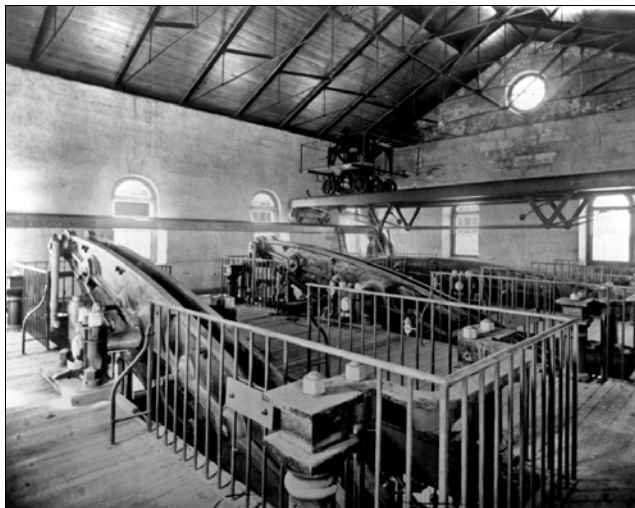
Upper floor of the Engine House, viewed from SW to NE., showing the 3 large, cast-iron rocking beams. The 3 steam cylinders are on the floor below, with steam pistons connected to the south (RH) ends of the rocking beams and pump pistons connected to the north ends Photo from Sydney City Archives, Sydney Water Collection A-00069858.
