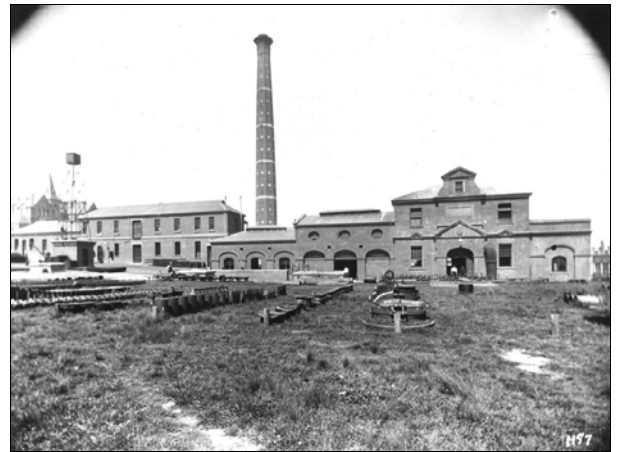
Crown St Reservoir is under the grass in the foreground, reservoir buildings in the background, and characteristic loads of plumbing fittings in rows on the grass. Over the years, the roof carried heaps of coal for the boilers, or large numbers of cast-iron valves, without any damage to the structure.
