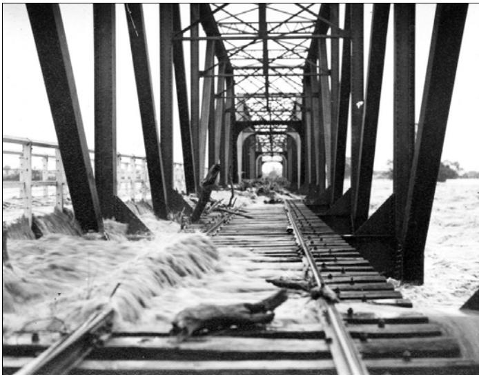
The 1950 flood at its peak. No record exists of who was intrepid enough to venture out onto the bridge at this time to take this photo. The view is from the south end of the bridge, looking north. The timber footway at left (upstream) was destroyed. Source: ARHS 122479.
