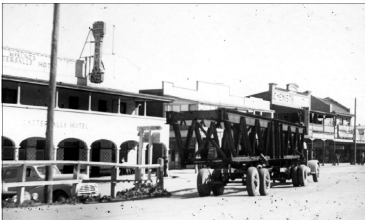
Image Left: A road jinker carrying one of the Warren truss spans through the main street of Kempsey, from Middleton Rd level crossing across the river to the Railway Station.
