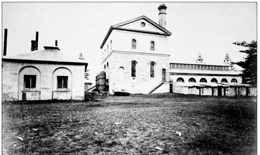
A different view of Botany Pumping Station, with Engine House (centre), Boiler House (right), and Workshops (left), viewed from the west c1896. Seen along the north side of the Engine House are the three iron air vessels, which cushioned the pulsed output from the pumps. Sourced from Water Board HRU Botany Sewage Farm File c1995.
