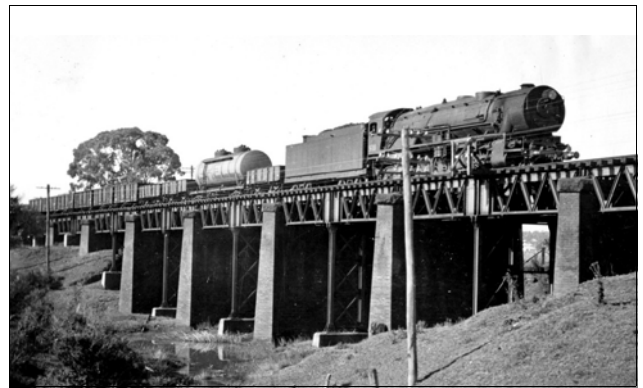
This bridge at Werrington on the Main Western Line is built with the same type of 1880s wrought iron Warren trusses as were re-used at Kempsey in 1950. These had been strengthened in 1920 with added mid-span trestle piers and web plates. This Werrington bridge structure remained in service until 1992.
