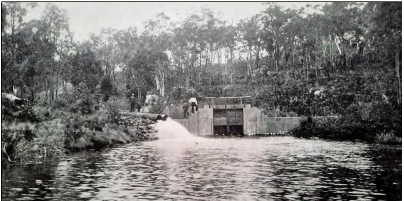
A 1900 photo of Victoria Reservoir. At centre left, two large pipes discharge clean water from the Clean Water Channel (see diagram above) into the Victoria Reservoir. At centre right, the wall is part of the Polluted Water Bypass (as above) – a diversion dam which captured the polluted run-off from the mills upstream of the Reservoir and diverted it around the edges of the Reservoir. Source: Water Corporation.
