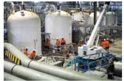
During peak construction time
