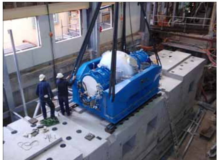
The primary refiner being lowered onto its massive foundation
