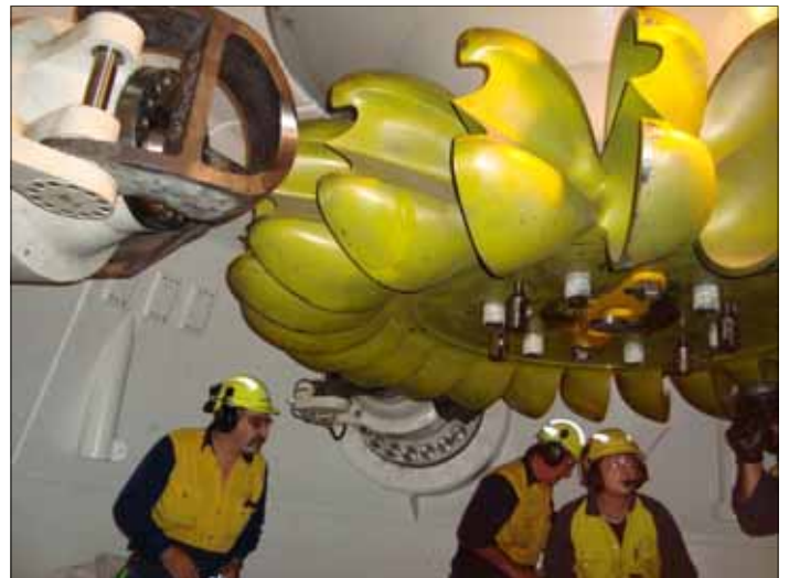
A runner being installed at Poatina powerstation
