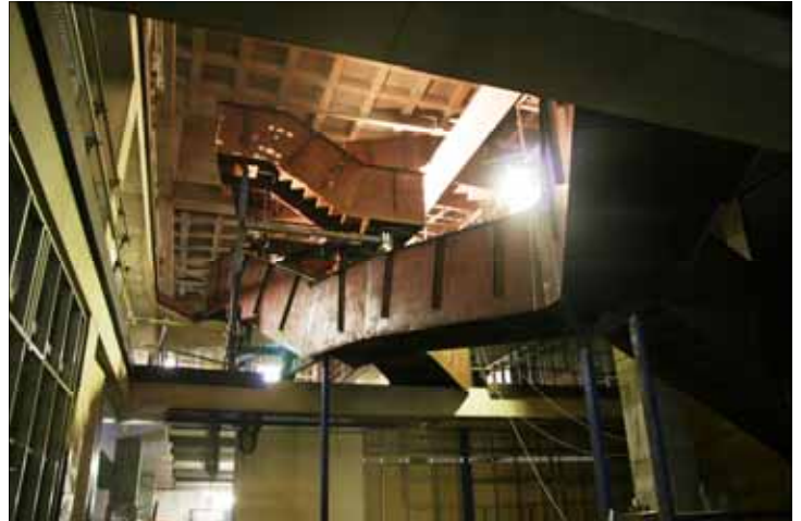
An impressive steel staircase within the complex
