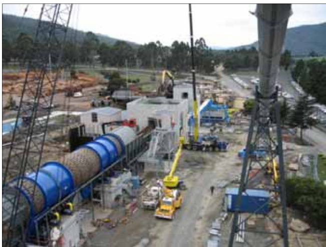
This photo shows the woodmill during the construction phase
