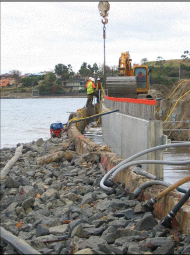
Precast wall panels being placed
