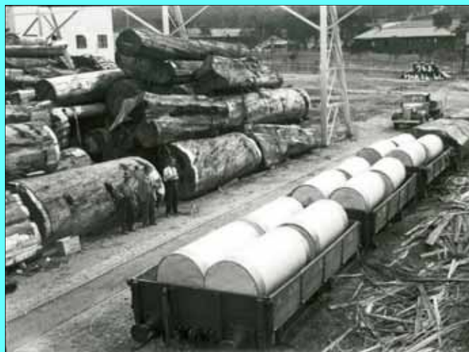
Rail wagons at the mill
