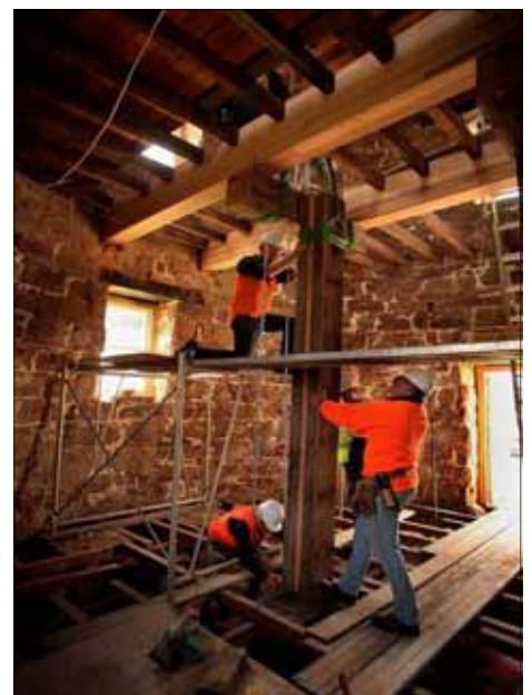
Restoration work in the tower
