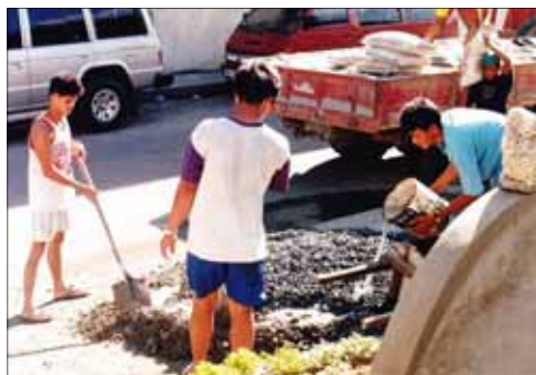
Mixing concrete - Concrete aggregate up to 75mm max size. Concrete batched by hand on the footpath. Note the safety boots !!!
