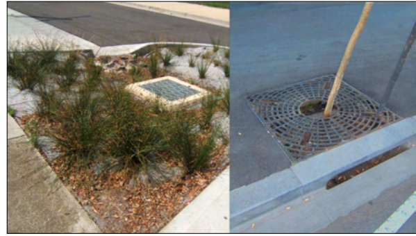
A biofiltration garden treating road runoff (left) and biofiltration tree-planters replacing standard stormwater entry-pits at Melbourne's Docklands (right)
