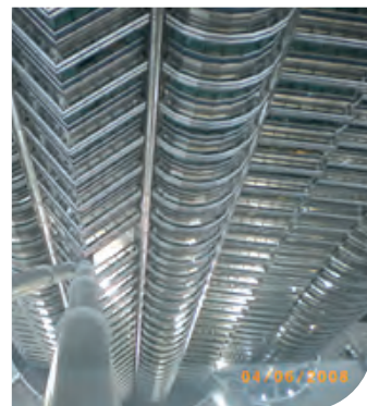
Reptile Skin, façade of the Petronas Twin Towers from the Sky Bridge. Photo taken by Nicolette Cumbo, Port of Melbourne Corporation.
