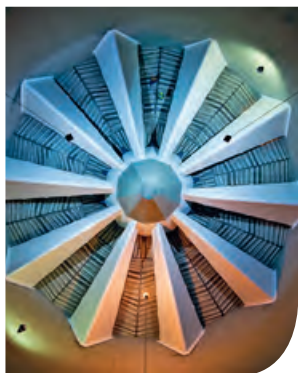
Melbourne Cement Facilities, Port Melbourne, photo taken by Dennis Kennedy – Director, Prostruc Consulting Engineers.
