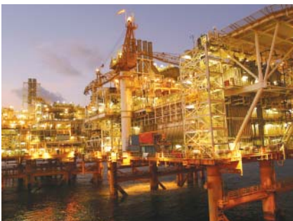
Above: Bayu - Undan Development, Phase 1 wins National Engineering Excellence Award
