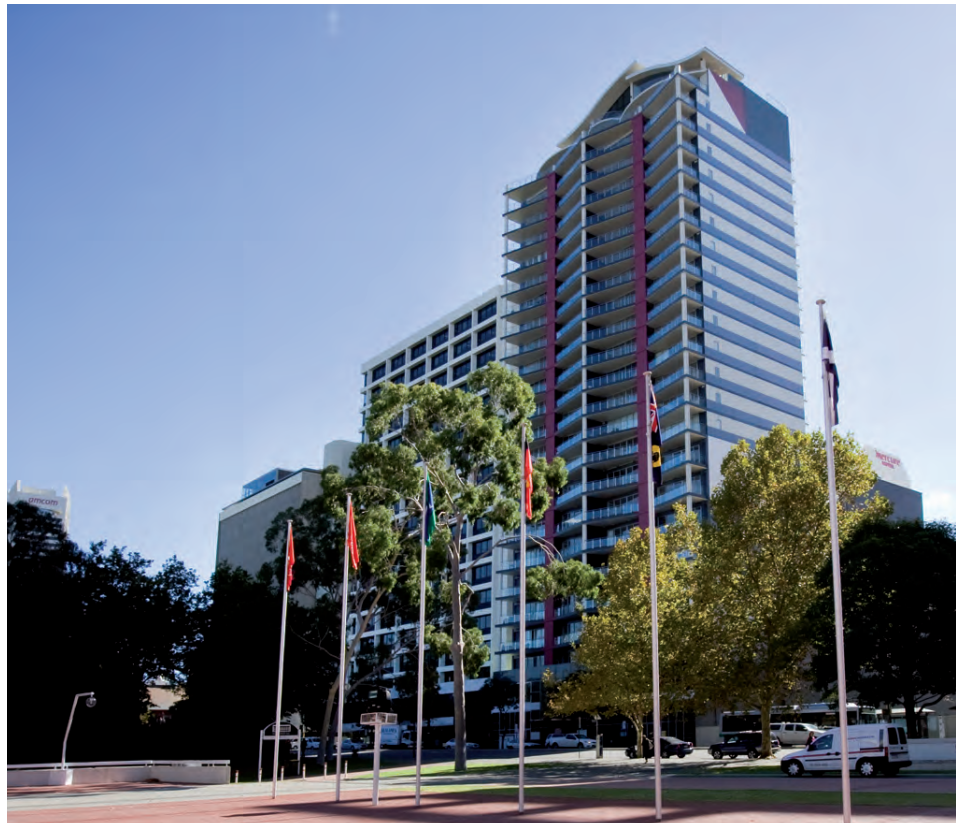
Above: Condor Tower, submitted by Pritchard Francis Pty Ltd, won the overall award as well as the Infrastructure & Building AND Innovation & Development Categories at the 2010 WA Engineering Excellence Awards
