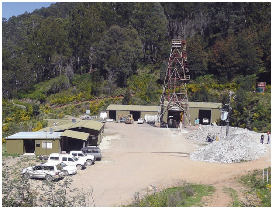
A gravity processing plant is to be installed at the Morning Star gold mine, which is to be restarted after being shut down for nearly 50 years.
