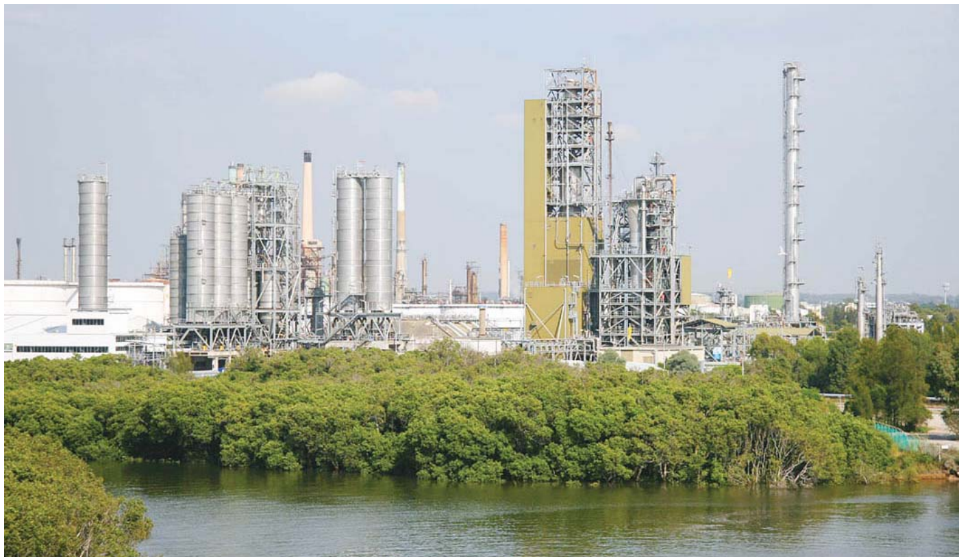
The new safety installation at Shell's refinery at Clyde in Sydney will replace several existing fire protection systems.
