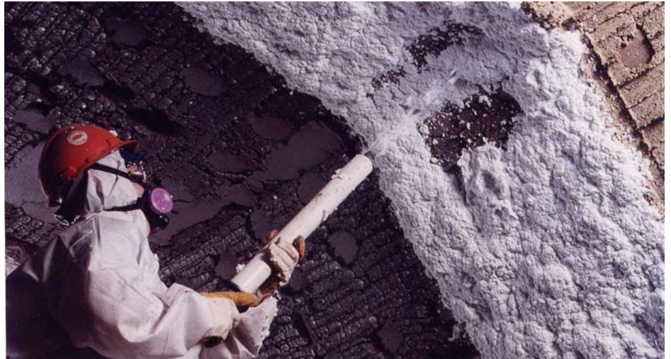
The Foamfrax insulation offers an alternative to brick, block and blanket furnace linings.
