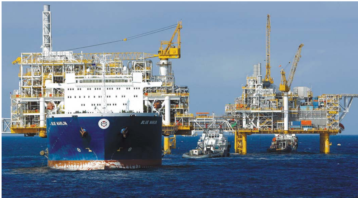
The Bayu-Undan gas recycle surface facilities in the Timor Sea's joint petroleum development area consist of three primary components: the central production and processing complex, the wellhead platform and the floating storage and offloading vessel.
