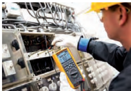
The multimeter diagnoses problems in plant equipment.
