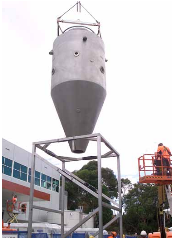
A 160t crane is lifting a drying chamber into a pharmaceutical processing facility in Sydney.
