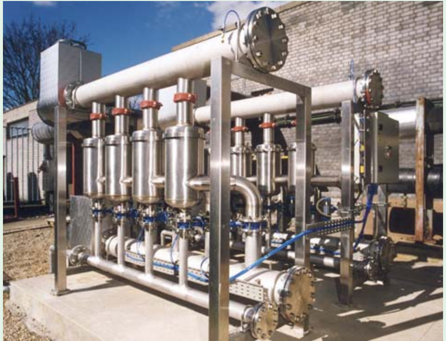
This automatic liquid filtration system is designed for high temperatures.
