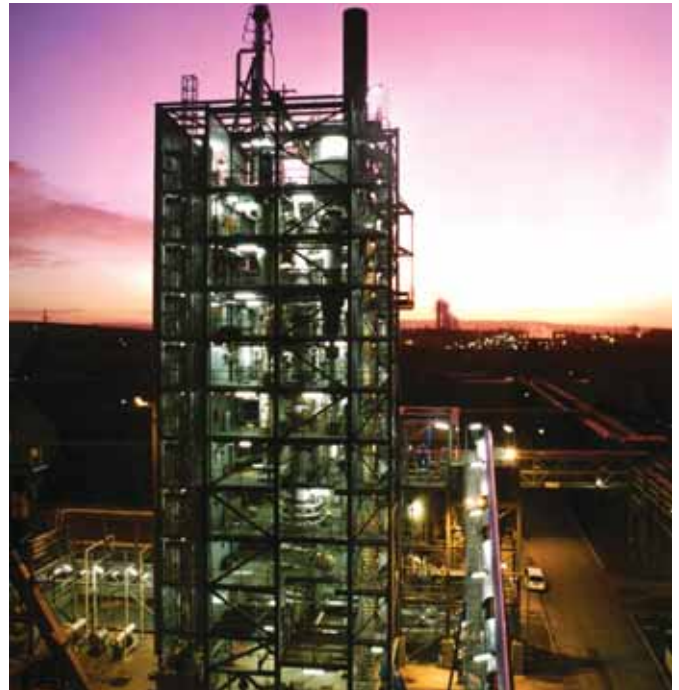
The 10MW gasification plant which was used to prove the integrated drying and gasification combined cycle technology.
