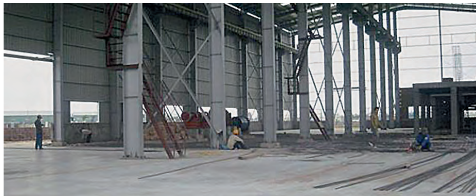
Ferrotungsten crushers will be installed in this furnace hall.
