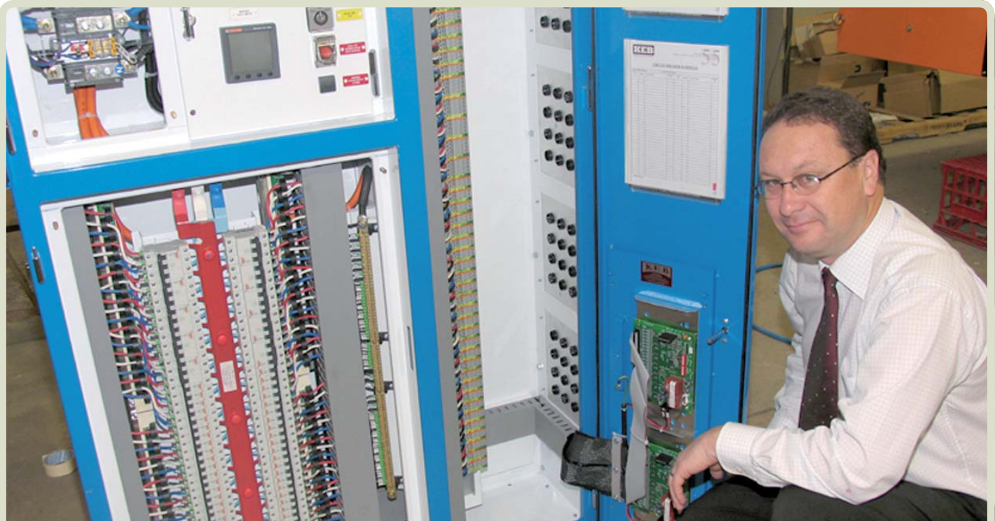
The circuit monitor helps safeguard security of data processing and industrial processing operations by determining the level at which current is drawn from individual circuits.
