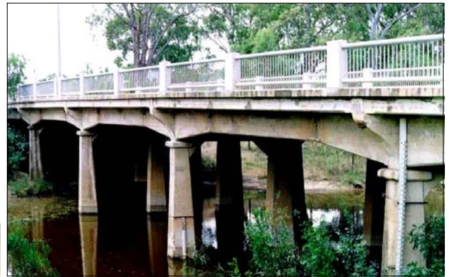
James Patterson Bridge in Charlton, photographed in 2010. All original work below the balustrade.
