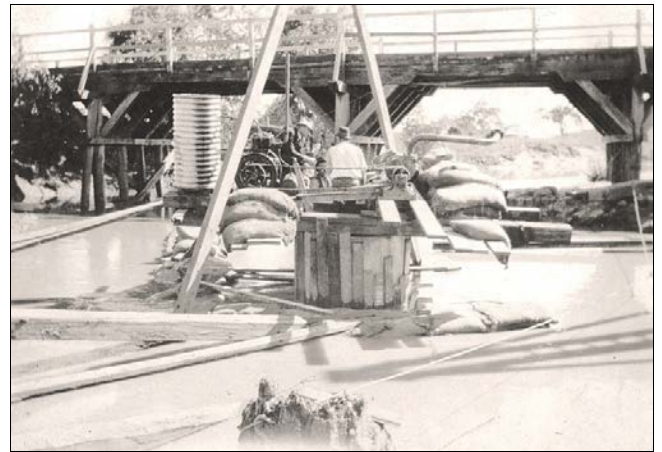
In-stream Pile Head Works, pre OH&S.
