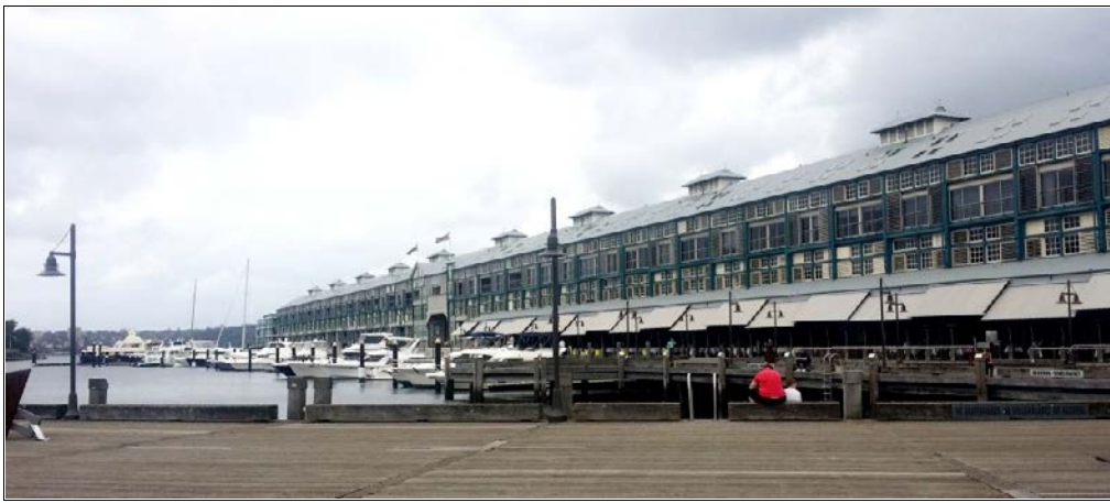
Wharf 9 (right) with awnings, wharf 8, and the new apartment building at the far end of wharf 8.
