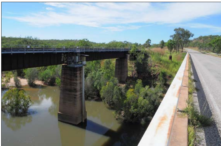
The Fergusson River Railway Bridge (1919) alongside the more recent Highway bridge. This railway bridge from the old North Australia Railway is the only one to be incorporated into the new Standard Gauge Adelaide to Darwin Railway. Photo: Owen Peake.
