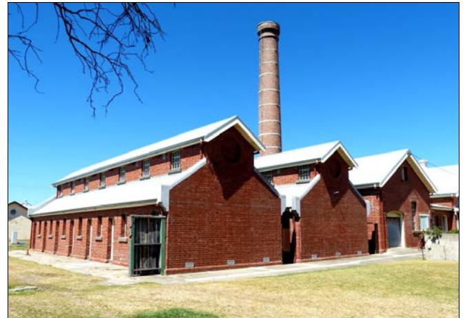
The 1899 twin Bath Houses and the adjacent Boiler House with its chimney. Photo: Keith Baker.
