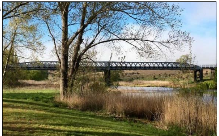
A beautiful bridge in its rural setting.
