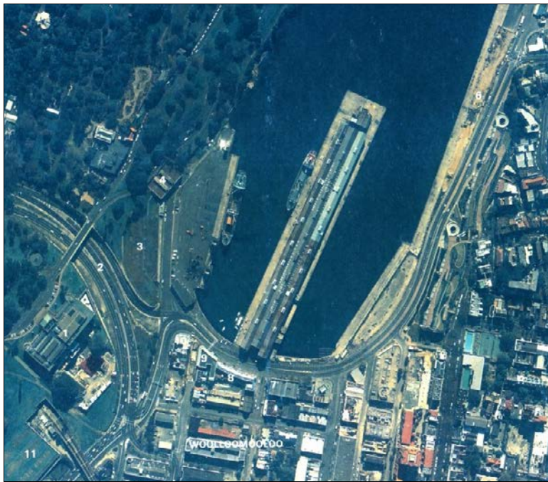
Aerial view of the Finger Wharf in 1987. The Art Gallery is on the lower left of the photo. The Navy Carpark is bounded by two white rings on the upper right side of the photo. Image: part of Exhibit 3.2 of the 1987 EIS.
