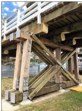
A rebuilt timber trestle.
