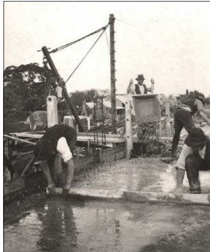
Concrete handling the hard way!
