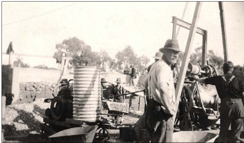
Concrete mixing 1920s style.
