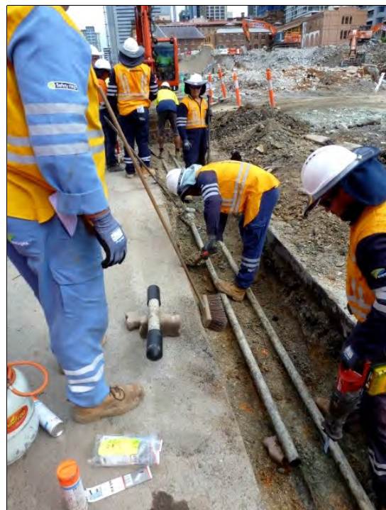
Left: The 2018 dig in William Street. Recovered Edison Street Tubes being cut and sealed for removal.
