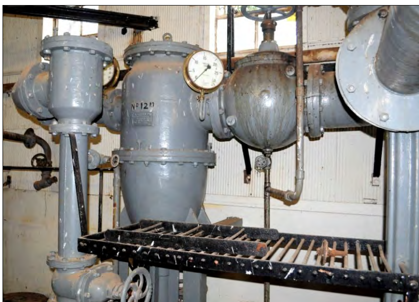
Image above: A Weymouth centrifugal pump with the top removed. Photo: Owen Peake.
