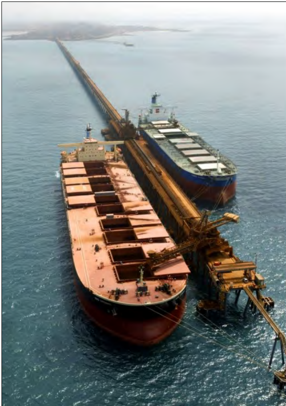
The end of the line. Not Dampier – this is where the ore from Robe River railway is carried by conveyor out to the ships at Cape Lambert port. Image - Rio Tinto.
