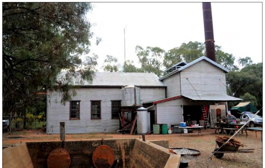
A view of the Millewa 'A' Pumping Station, showing the pump delivery pit in the foreground. Photo: Owen Peake.
