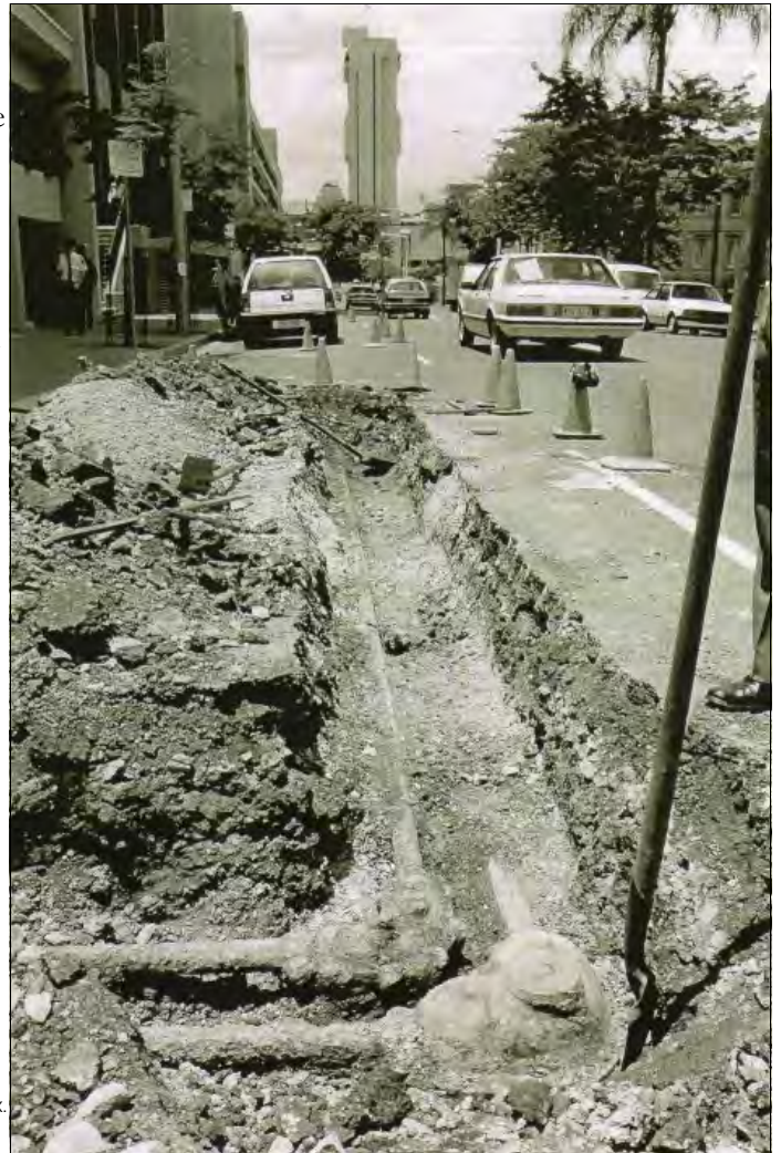
Left: The 2018 dig in William Street. Recovered Edison Street Tubes being cut and sealed for removal.
