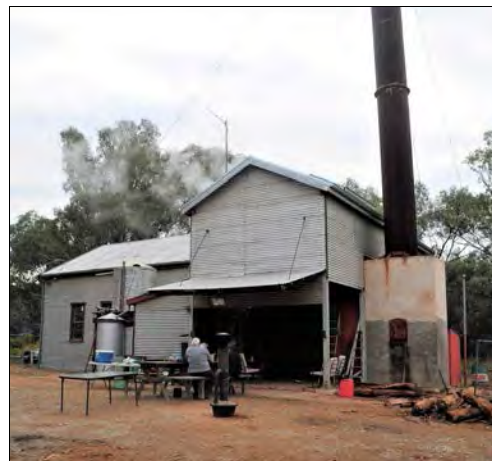
Millewa 'A' Pumping Station. Photo: Owen Peake.
