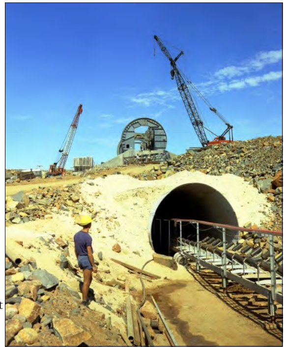
Rail-car dumper under construction at Parker Point, Dampier in 1966. The dumper (top centre) would tip the ore from Mt Tom Price ( see image previous page) into the conveyor emerging from the tunnel at right. Image - Rio Tinto.
