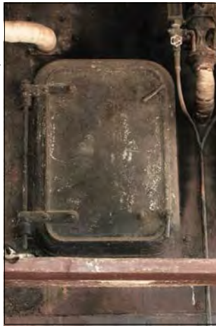
Closed top left boiler door. Part of photo on page 16.
