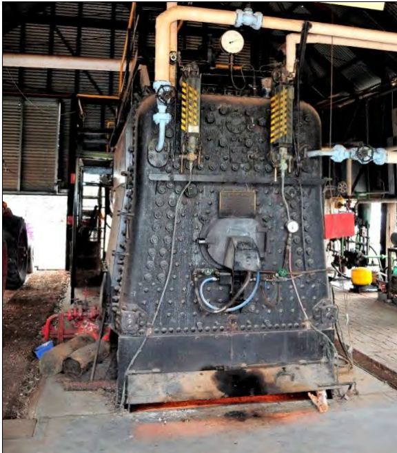
The Psyche Bend Boiler in operation on the day of the ceremony. Photo: Owen Peake.
