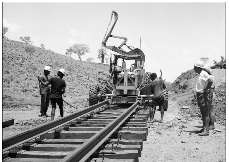
Above left & right: Thursday Islanders laying track, 1965/66.
