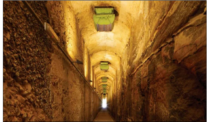
The interior of one of the tunnels, showing the coal chutes in the roof, through which the coal was poured into the travelling feeders, running on rails mid-height on the side walls.. Photo: Landscape Architecture Australia. 2016
