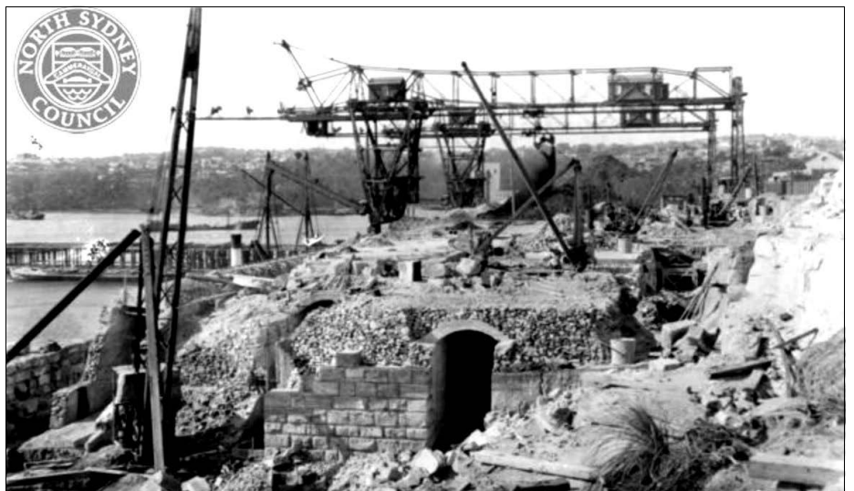
Construction of tunnels 1-4 and the south sandstone wall, Balls Head Coal Loader, 1918. Note the incoming coal unloading gantry cranes already in situ, and probably in use unloading building materials from the ship lying alongside the wharf. The coal outloading pier is under construction in the background.
