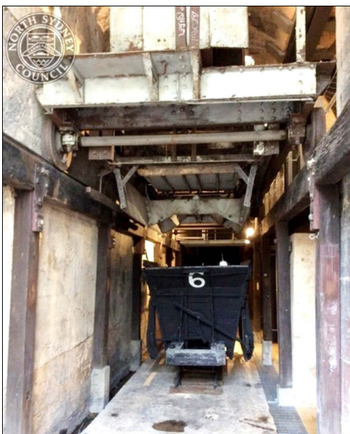
Image at Left: The base and underside of a surviving travelling feeder, perched under the roof of Tunnel No.1 on its wheels, ready to roll along the rails fixed to the sides of the tunnel. The hopper No.6 on the floor under the feeder, is one of only two surviving after the closure of the coal loader. It was restored by ICS some years ago. Photo: by David Banbury, 2018. Source: NSC.
