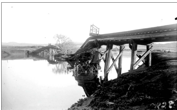
A view of the destroyed trestle bridge after the flood of July 1922. Source: NAA A3560, 228.
