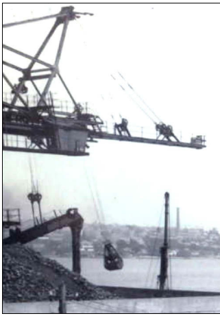
Part of a 1920 photo with a loaded grab bucket about to dump its coal on the stock pile, Source: Bonzle.
