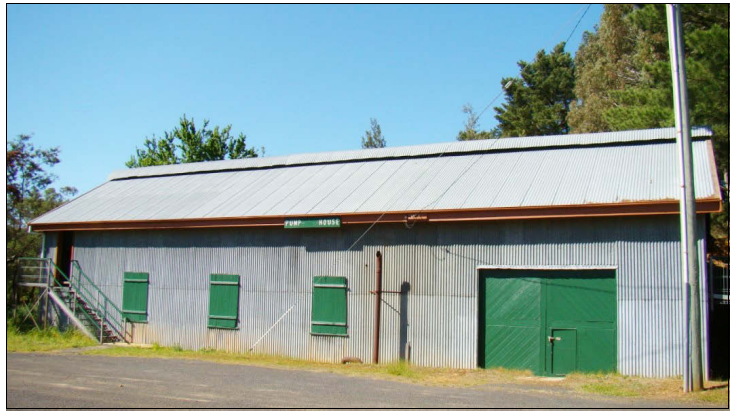
The Lake Canobolas Pump House. This view is of the side of the building facing the dam wall. The Producer Gas Plant is behind the double doors at right. Source: Orange Council.
