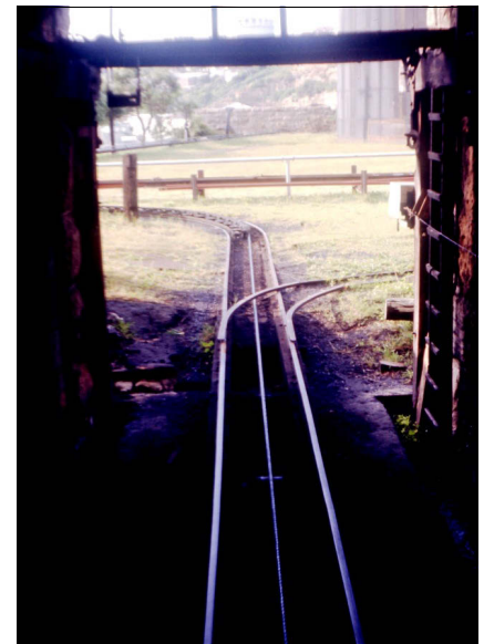
Cable tramway rails and cable emerging from a tunnel and turning left towards the pier. A maintenance siding curves off to the right.
