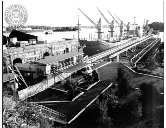
The Coal loader in its final configuration, with the coal moved by high-speed conveyor belts instead of hoppers moved by an endless cable. This photo shows the ship " High Adventure " docked at the pier for loading. This system was installed and operated by Coal and Allied Industries. Photographed circa 1990 by Robert Donnell.
