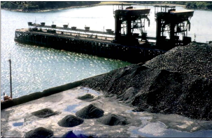
Part of a 1960s photo of the coal deck and the outloading pier. Shows (lower left) 2 of the holes in the deck above tunnel No.1 down which the coal is poured to the travelling feeder below. Top half of the photo shows the pier with the outloader structures and a number of hoppers lined along the cable tramway.
