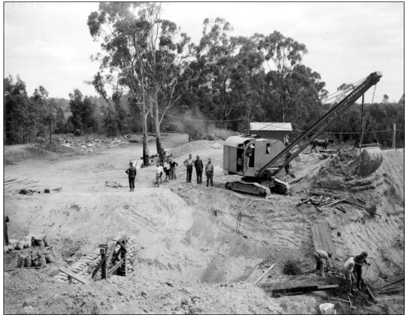
Flood reclamation works on a drainage channel using a Harman dragline (1934). Source: State Library Victoria.
