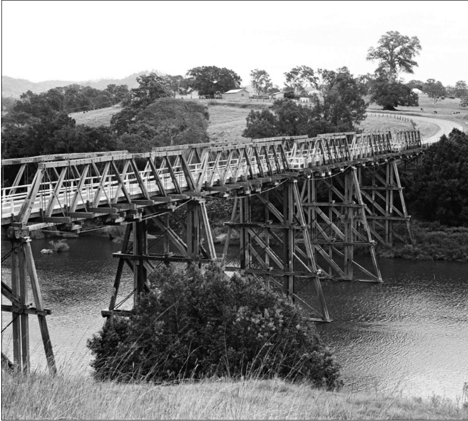
Killawarra Bridge 1983. Photo - M Doring.
