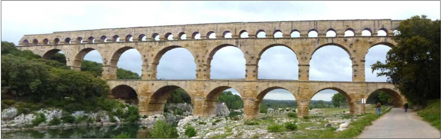
The Pont du Gard, a 3-level stone aqueduct crossing the Gardon River between Uzès & Nîmes. Built 19 BC for the Emperor Augustus. Photo Peter Haughton This view of the south side of the bridge was taken from the right bank, looking north (upstream) towards the tourist centre on the left bank. The 1743 (new) lower level & roadway is on the other (north) side of the bridge from this photo.
