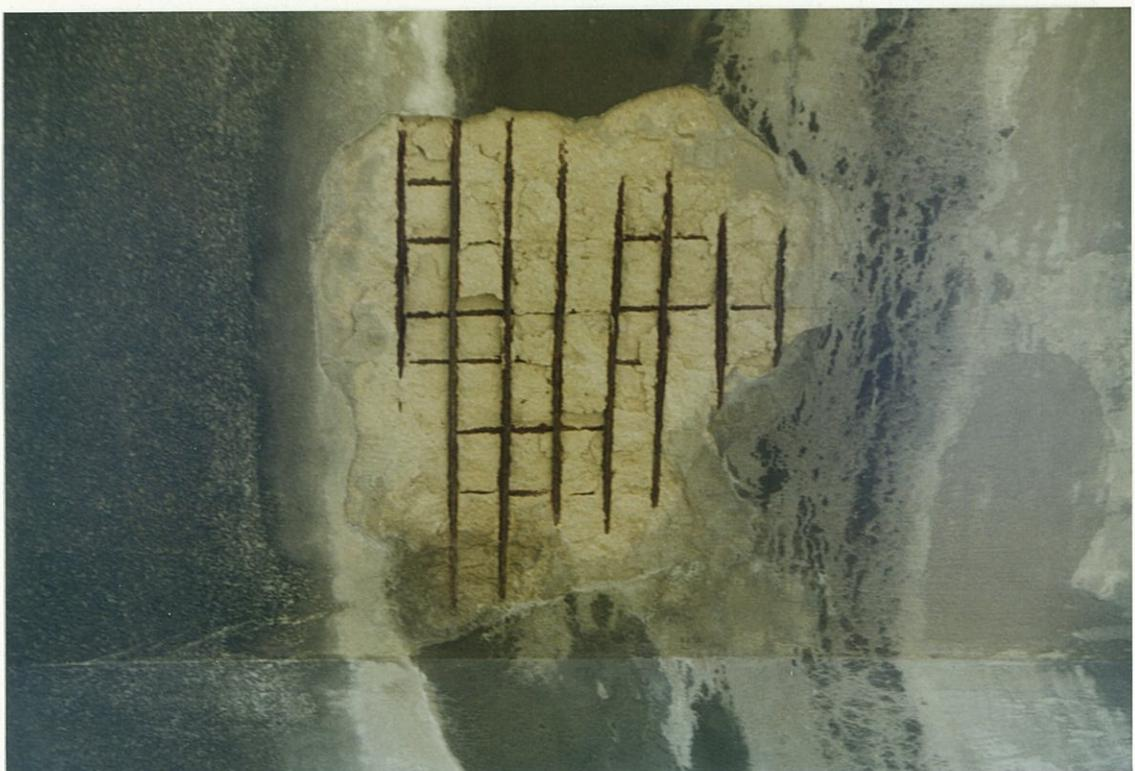
*Exposed reinforcing mesh on the soffit of Johnstone's Creek sewer aqueduct*
