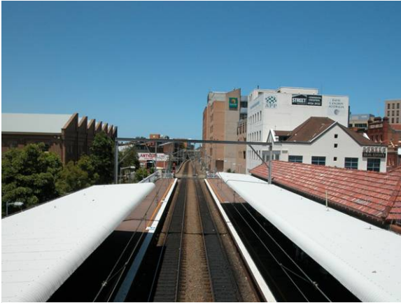
Photo 1: Looking east from the present Civic Station, previously the site of the original Honeysuckle Point Station. The original line ended at the street boundary of the level crossing in the middle of the photo. The saw-tooth roofed building on the left forms part of the Honeysuckle Workshops (HEM 1996).
