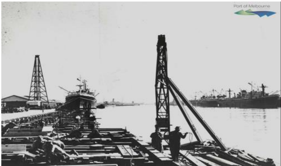
Workers during the construction of Victoria Dock.
