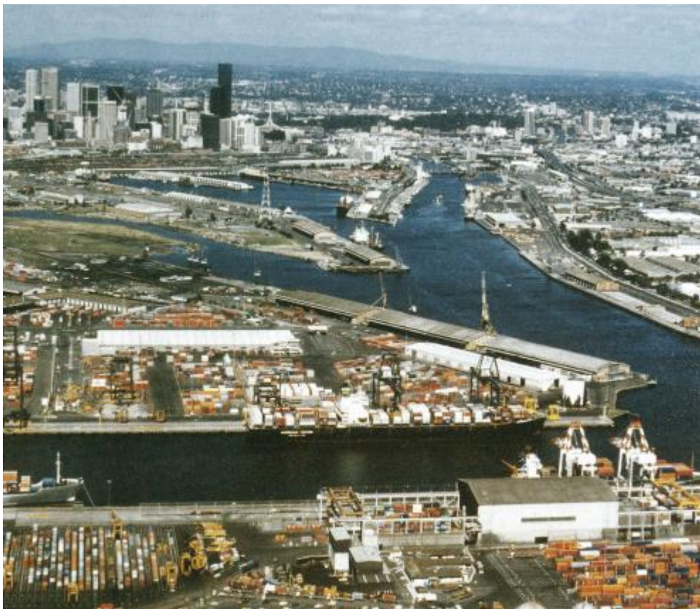
Aerial view of the Port of Melbourne in the 1980s with Swanston Dock in the foreground. Image: Public Records of Victoria.
