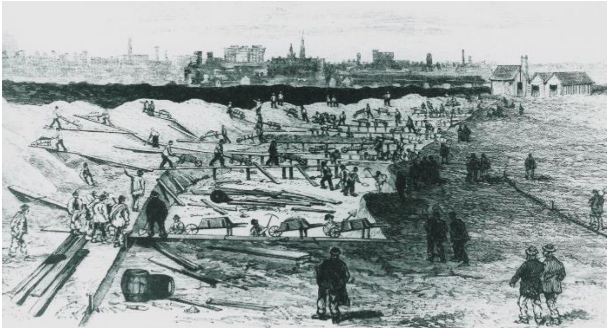
Image of excavation works at Fisherman's Bend during the digging of the Coode Canal (1889). Image: Public Records Office Victoria.
