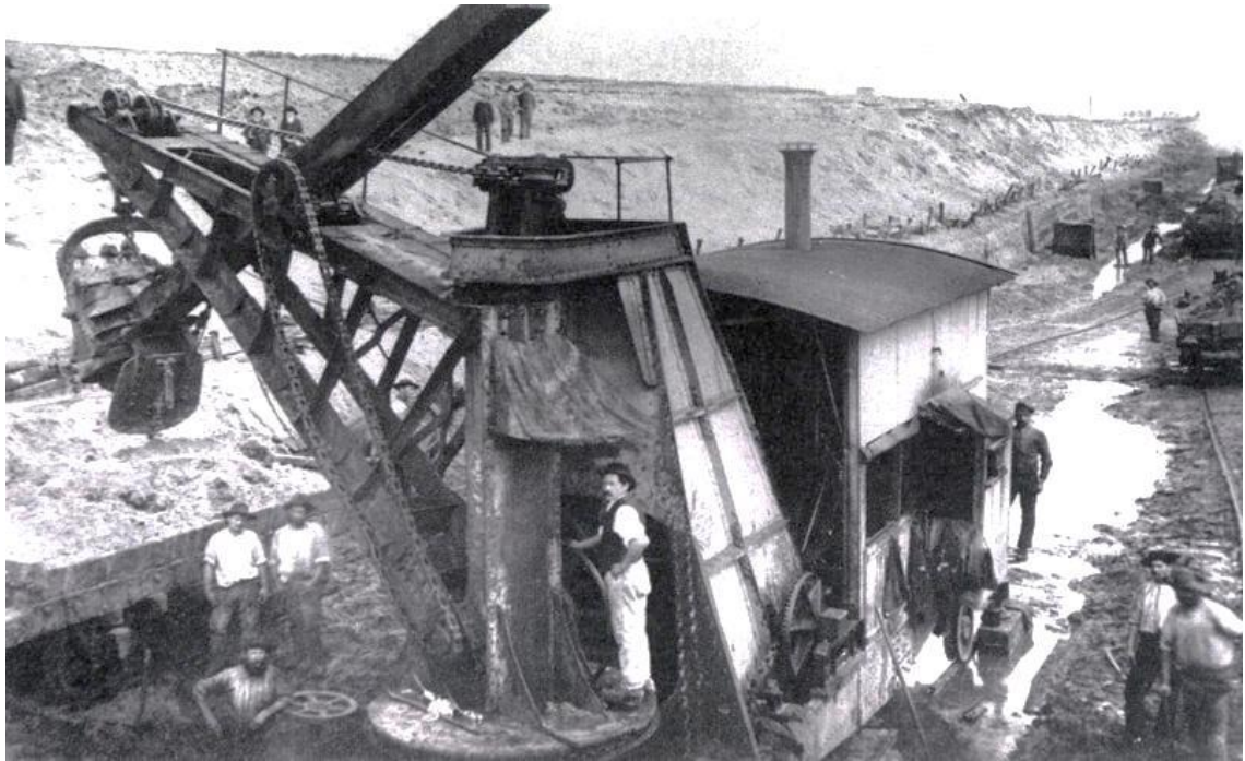
Steam driven machinery being used to create the Coode Canal during the 1880s.
