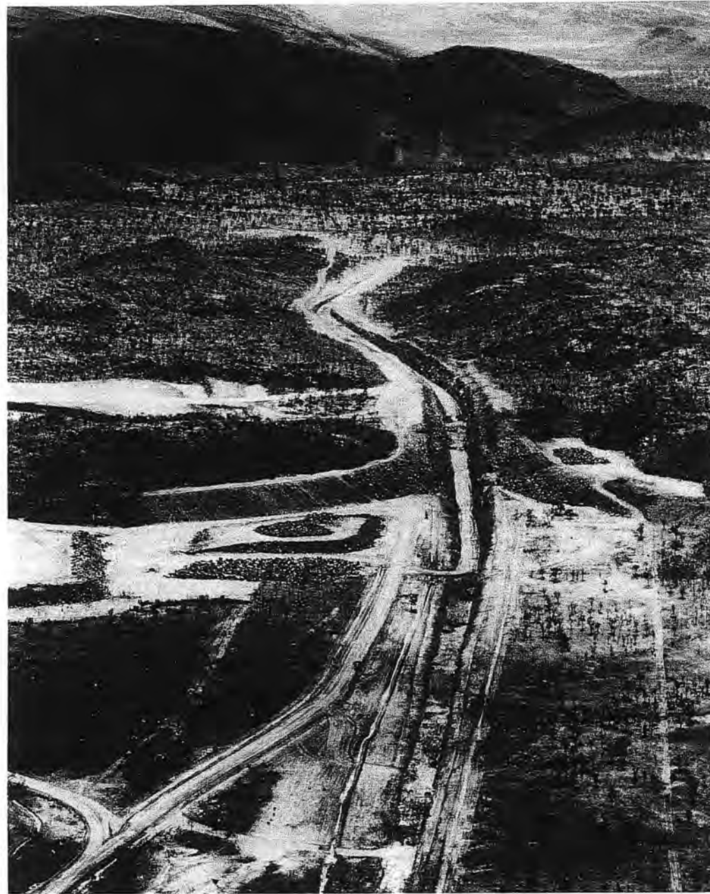
Spillway Channel viewed from upstream
