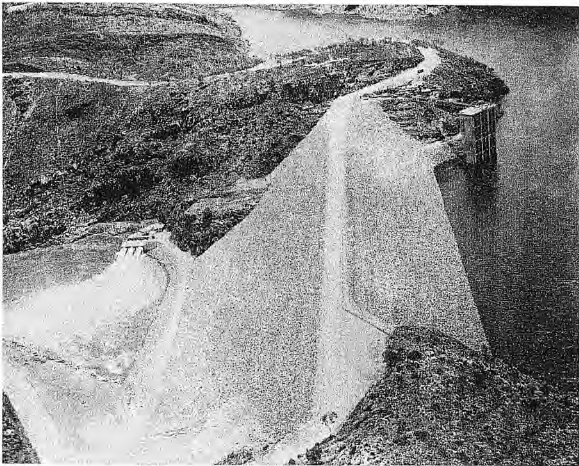
Fig. 1.—View of Completed Dam.
