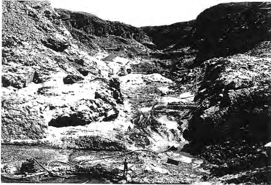
Foundation excavation nearing completion, June 1970
