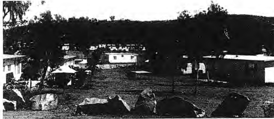
The Contractor's housing
