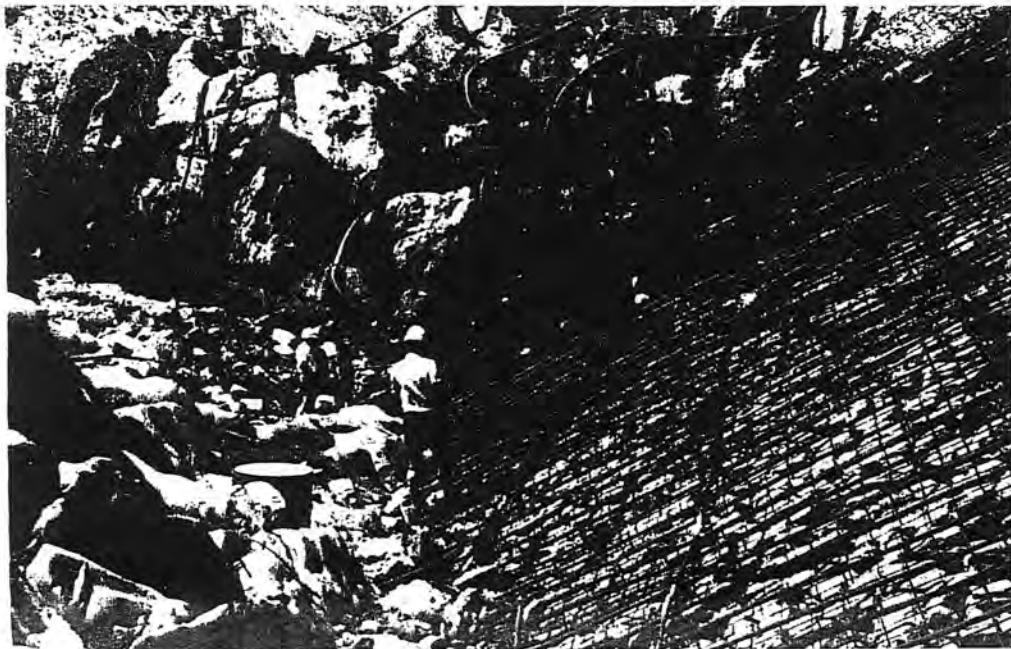
Protective steel mesh at downstream toe of the embankment
