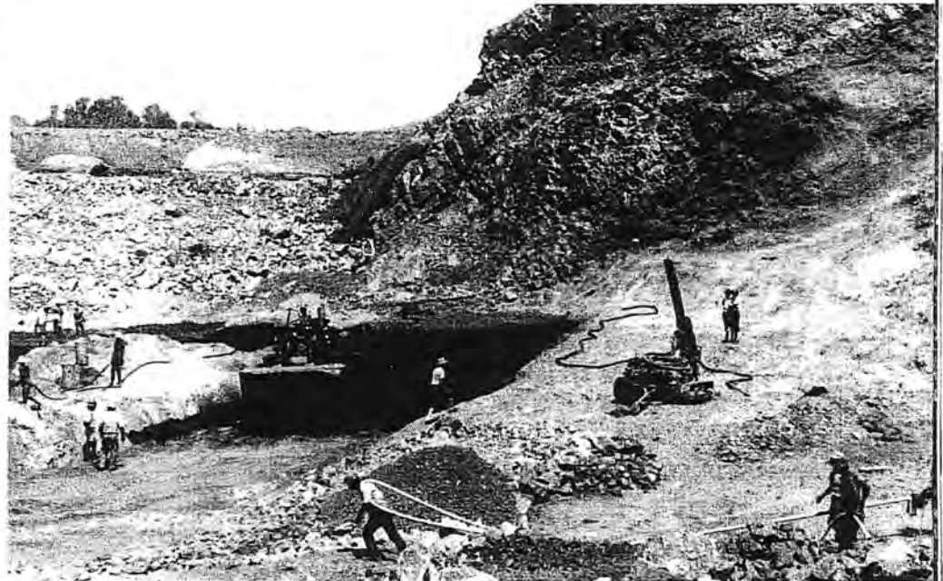
Placing clay core in foundations, September 1970
