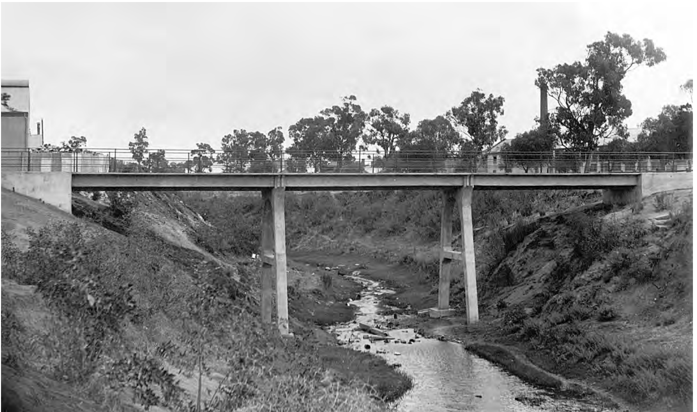
The Holland Street Bridge soon after completion (looking west) – “architecturally creditable” [University of Melbourne Archives, BWP/23733 Reinforced Concrete & Monier Pipe Construction Co]
