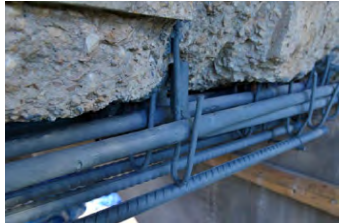
(Left) Original bars were bent-up to provide shear reinforcement near the supports – note corrosion of bows (Right) Examination of the reinforcement shows where the bar is slightly wider than it would have been when it was rolled – the forge welding been very well done and might not have been noticed without the evidence of Monash's letter to Harvey (note the modern reinforcing below which is part of the reconstruction project)
