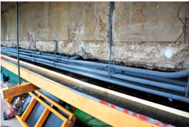
(Left) Formwork in place for the trial beam repair: loose concrete has been removed, the old reinforcement primed, and new reinforcement placed
