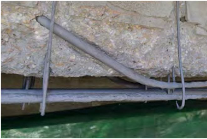
(Left) Original bars were bent-up to provide shear reinforcement near the supports – note corrosion of bows (Right) Examination of the reinforcement shows where the bar is slightly wider than it would have been when it was rolled – the forge welding been very well done and might not have been noticed without the evidence of Monash's letter to Harvey (note the modern reinforcing below which is part of the reconstruction project)
