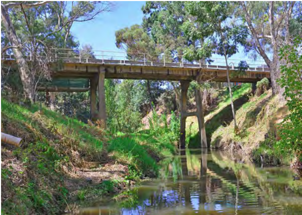
The Holland Street bridge during the trial repair in 2013 – the access scaffold used by the contractors can be seen on the left [Photo: John Woodside]
