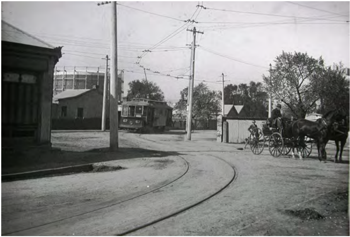
Hindmarsh-bound [Type X] tram No 67 negotiating the dogleg from Albert into Holland Street in 1910 Note the use of plain wooden poles in the side streets – compare this with the ornate steel poles in Manton Street, page 19 [Photo: John Radcliffe]
