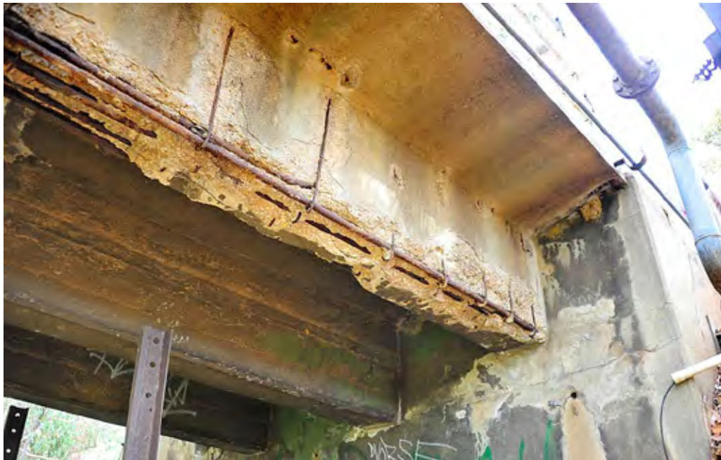
The outer beam on the eastern side in 2011 – this was the worst-affected beam and the one chosen for the trial repair [Photo: John Woodside]
