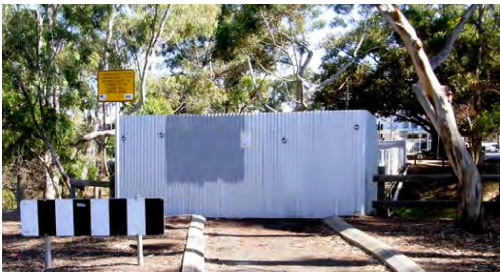
The bridge viewed from Holland Street after its complete closure in 2011 [Photo: Richard Venus, 15059]
