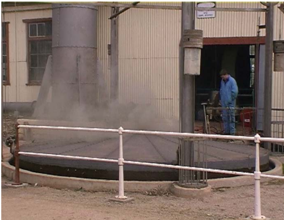
Photo 4: The top of the water tower, which sits below ground. The water in this tower rises and falls as the pump operates.
