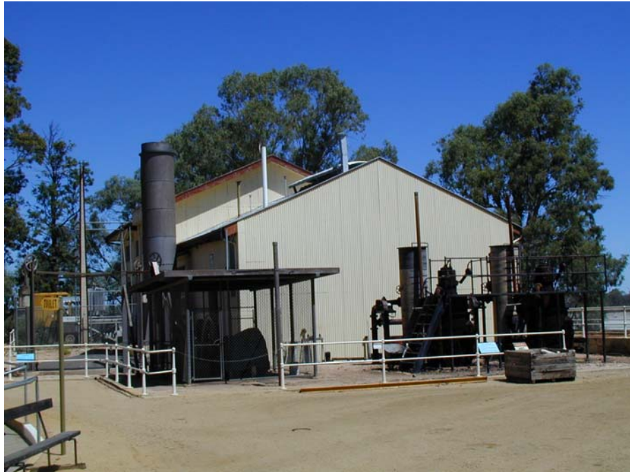
Photo 1: Cobdogla pumping station which houses the Humphrey pumps.
