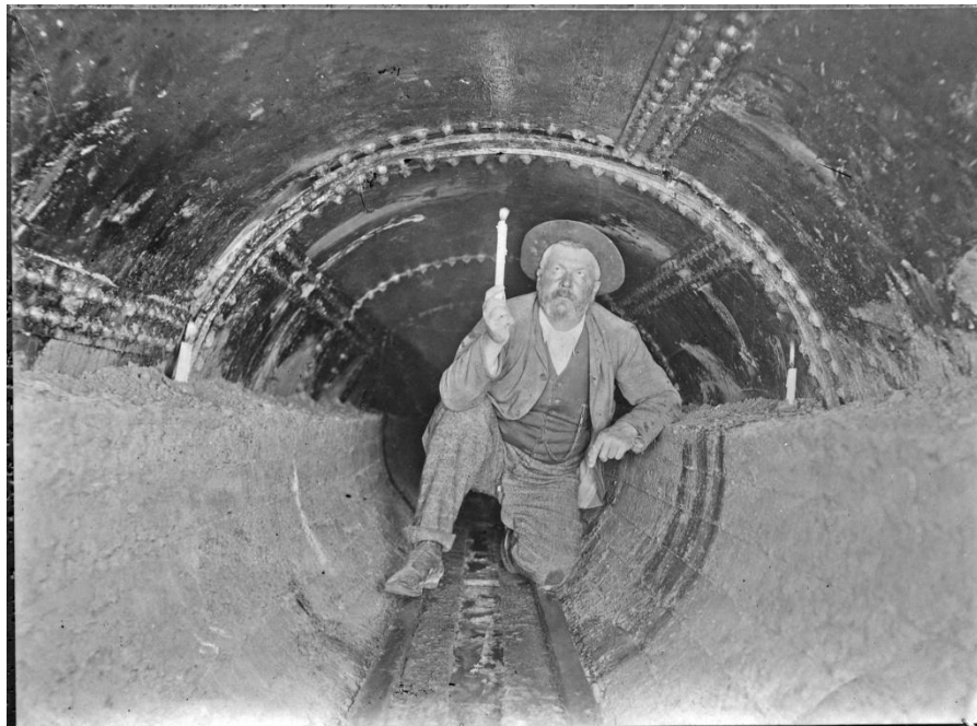
Inspection of the rising main from Spotswood to Brooklyn where the Main Outfall Sewer started. It was ultimately corrosion in this main which led to the closure of Spotswood Pumping Station. Image: source unknown
