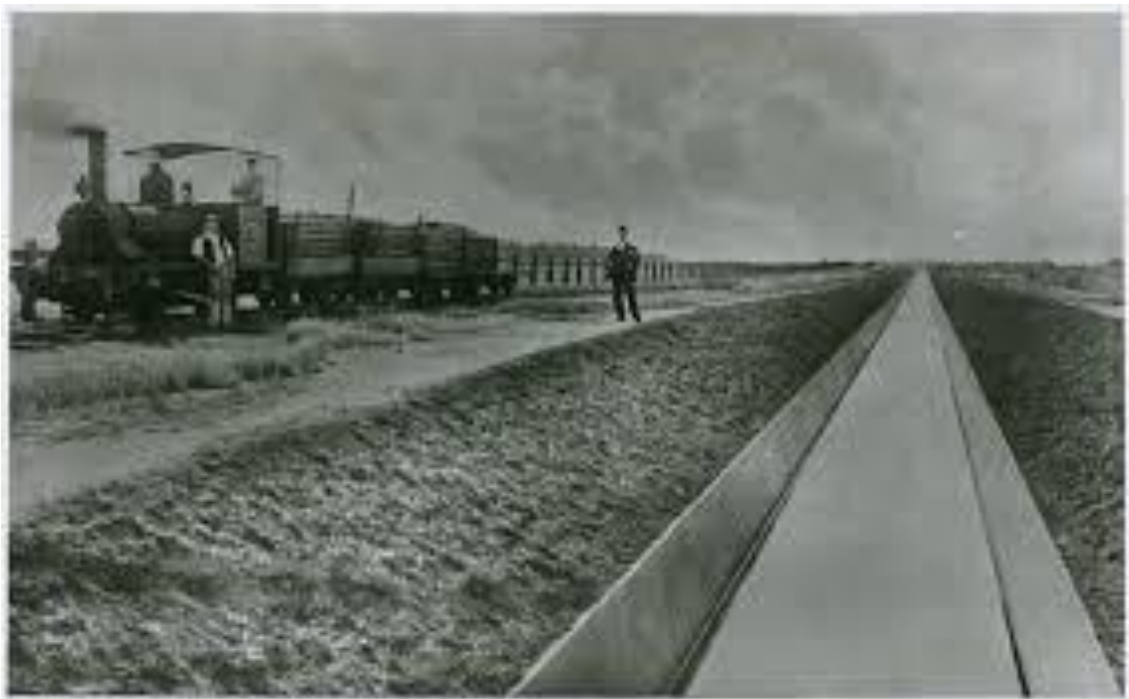
Main Outfall Sewer. Image: Culture Victoria
