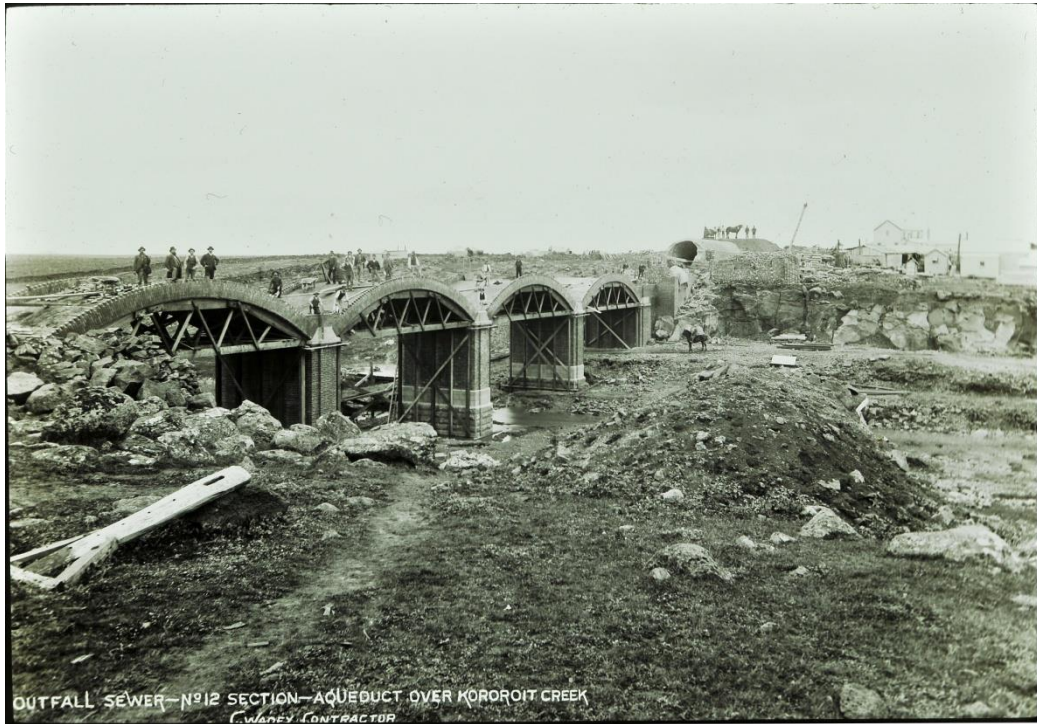
Kororoit Creek aqueduct for the Main Outfall Sewer. Image: source unknown
