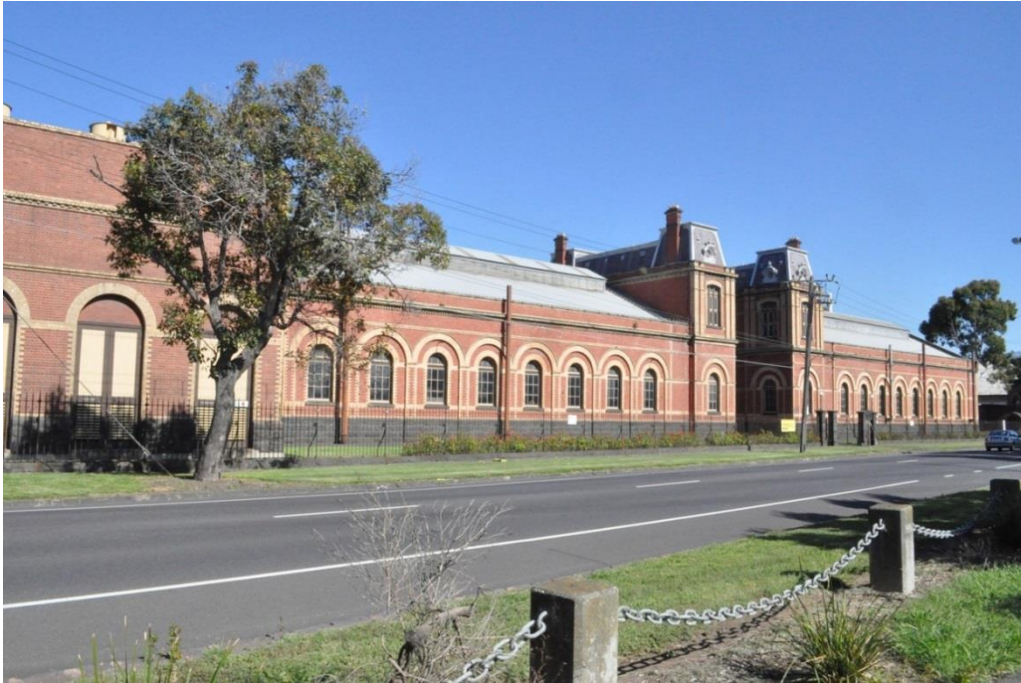
Spotswood Pumping Station from the river bank, 2011. Image: Owen Peake
