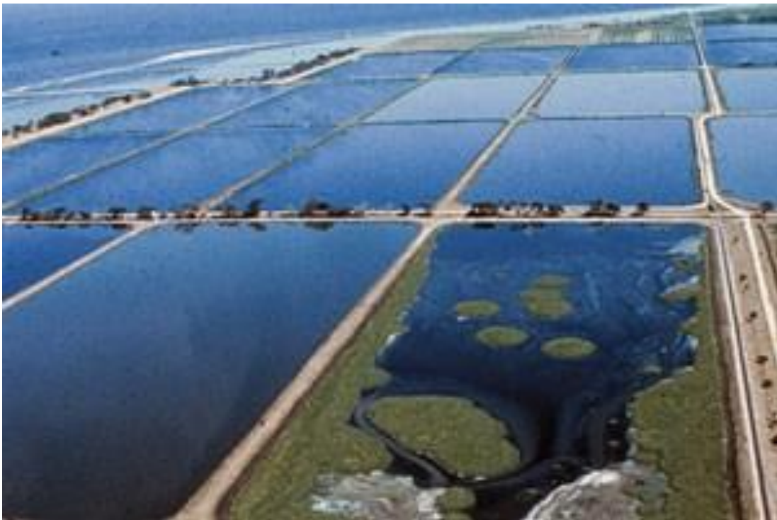
Oxidation ponds at Western Treatment Plant. Image: Melbourne Water
