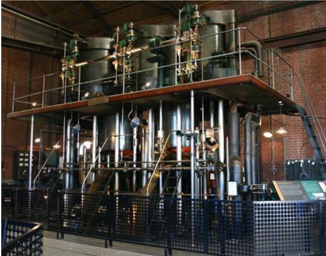
Steam Pumping Engine - Austral Otis, No.8 Pumping Engine, MMBW Spotswood Sewerage Pumping Station, 1911 (ST 038266). Source: Museum Victoria
