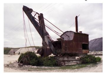
Cement Company between 1925 and 1980 mainly excavating limestone. It is presently disassembled, and is the sister shovel to one on display at the Lake Goldsmith Steam Preservation Society. These two shovels are the largest surviving steam powered shovels in Australia. The photo shows the shovel on the quarry floor in 1992. The shovel is significant for its use of steam power, its intactness and size, and its long documented working history at the quarry.
