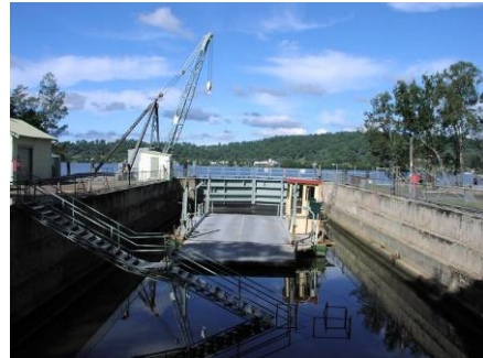
Ashby Dry Dock
