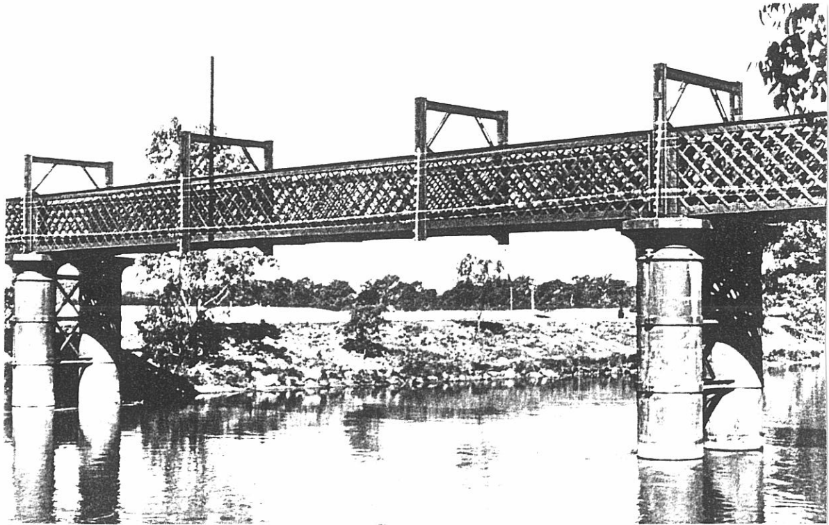
A river span of the lattice bridge which shows the 1929 sway frames.
