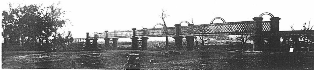
The lattice girder bridge prior to reconstruction of the viaducts. Note speed restriction lamp at approach to bridge.
