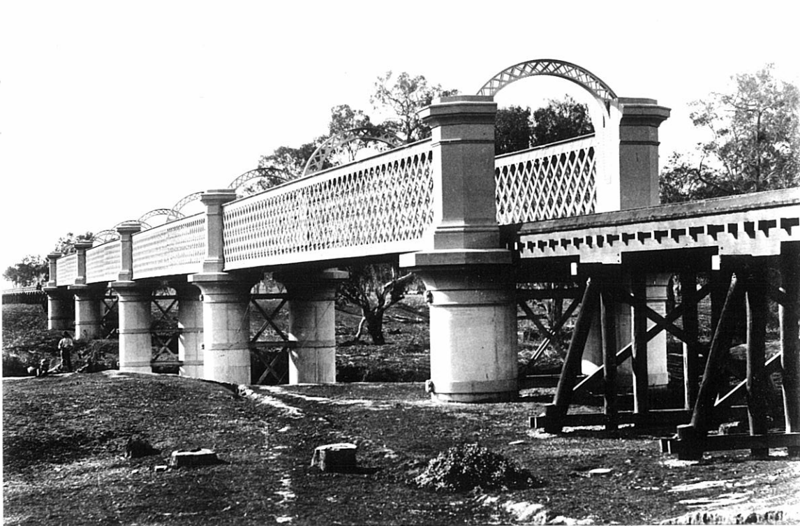
The lattice wrought iron railway bridge and the original timber viaduct c1890
