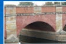
View of arch showing details of brickwork
