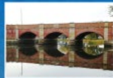
View of Red Bridge from downstream
