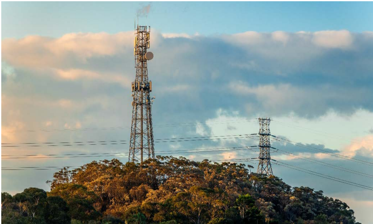
There is a growing dependency between energy and telecommunications
