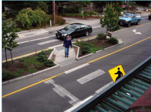
Photo Credit: Bruce Landis, Angled cut-through in Bainbridge, WA
