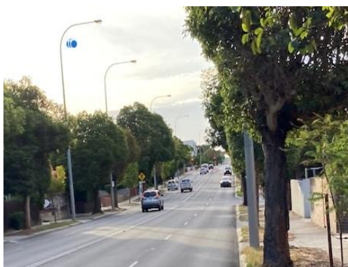
Four-lane undivided road
