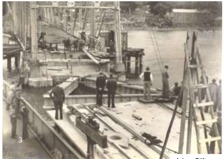
Joining bridge to lift span
