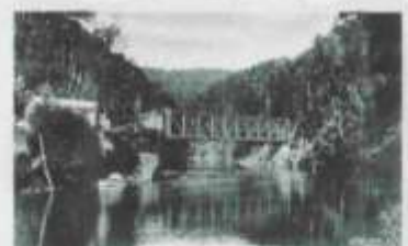
The bridge was built in 1884 and is made of iron. It was built by the engineer E. C. De Pater.
