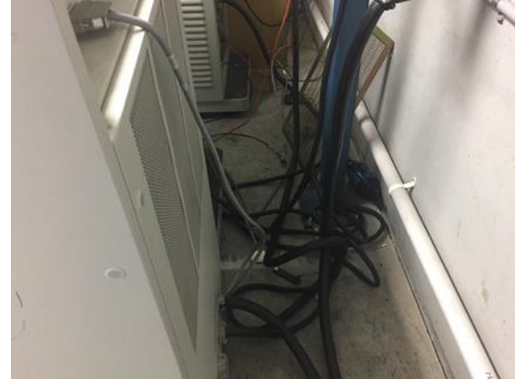
Fig. 3. Long interconnecting cables can cause errors.
