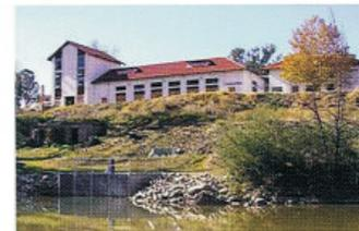
Canberra's population. The building architecture changed in 1963 so that motors and electrical gear for the additional pumps 7 & 8 could be installed on the upper floor, above the level of a major flood, but remained consistent with the Murdoch style.
