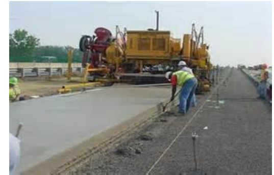
Slip-formed Concrete
