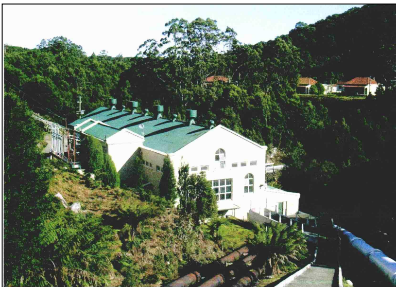
Lake Margaret Upper Power Station
