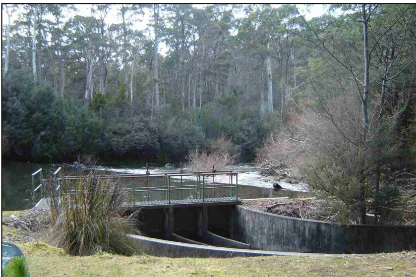
Weir and Intake at St Patricks River
