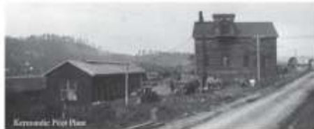
Kermadec Pilot Plant
