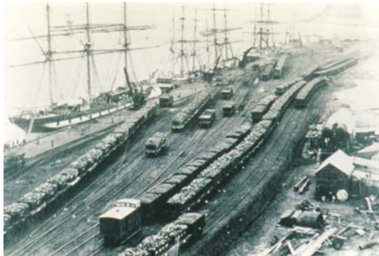
Queen's Wharf, 1875. A number of the concrete bases for the steam cranes can still be seen.
