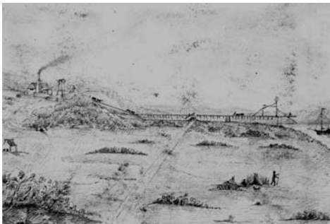
A depiction of the AA Company 'A' Pit, from 1831. Some remains can still be seen on the walk.
