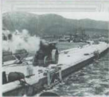
Transport links accelerated Tasmania's social and economic development. The floating bridge across the river Derwent allowed Hobart's western shores to develop. The Museum's rotary traction engine was utilized for construction of the innovative bridge in 1893.
