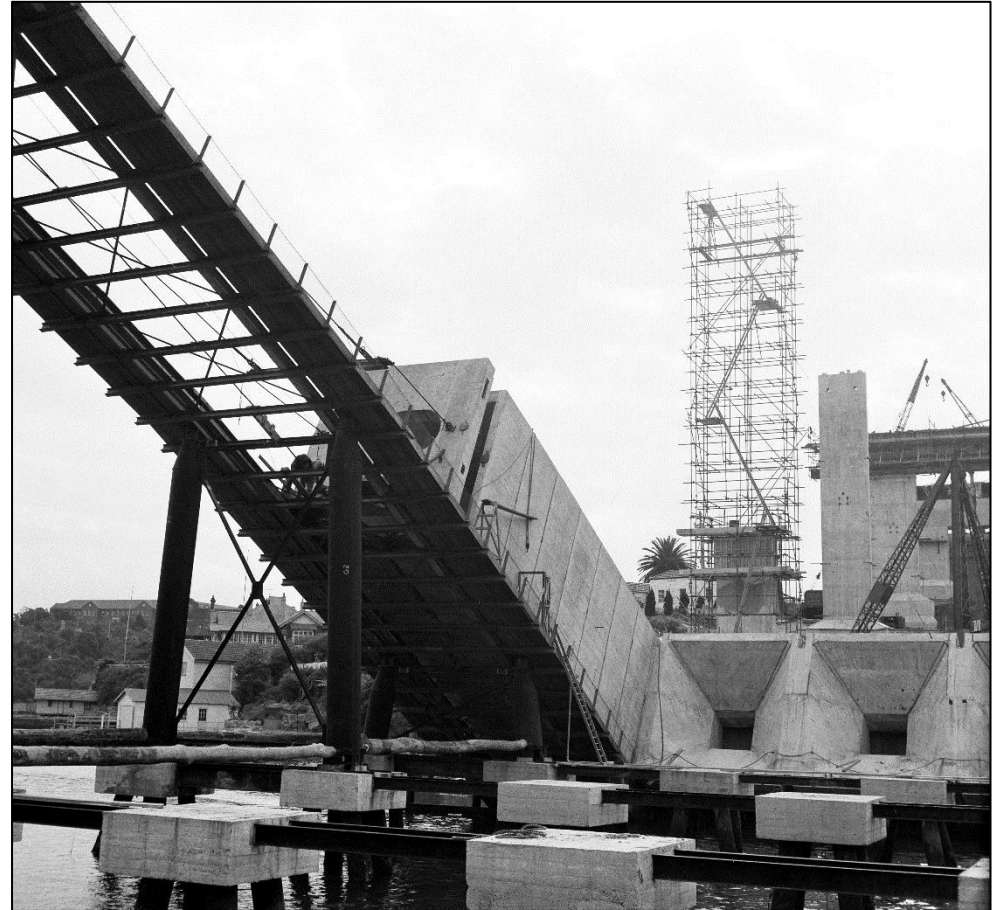
Installation of Precast Diaphragm Unit
