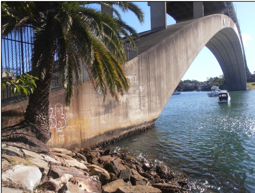
Drummoyne Abutment (June 2014)
