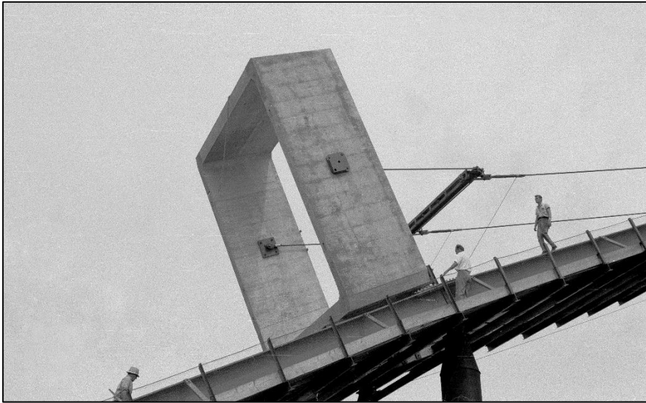
Precast arch unit winched along falsework on trolley
