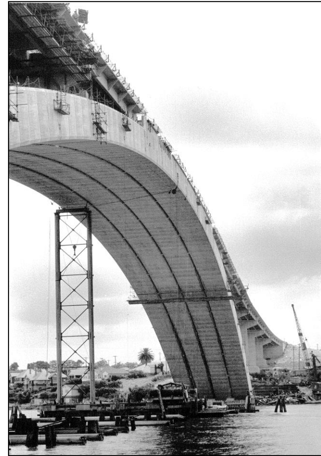
Self-supporting arch ribs
