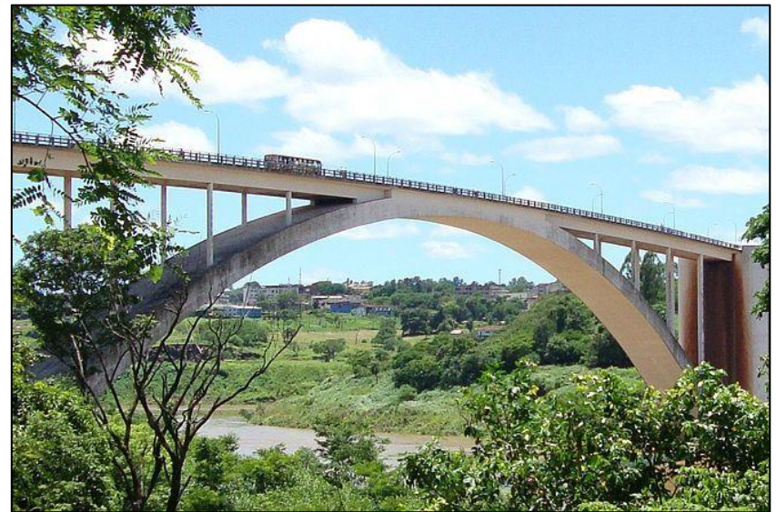
Iguacu Bridge (Brazil/Paraguay border) – opened 1965, arch span 290m
