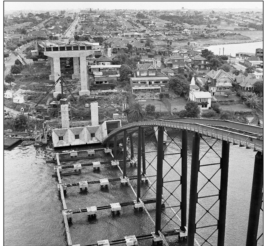
Drummoyne end of bridge
