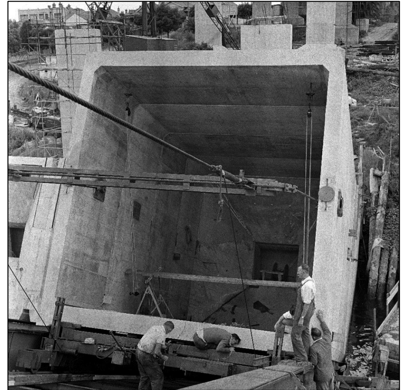
Final placement of precast arch unit
