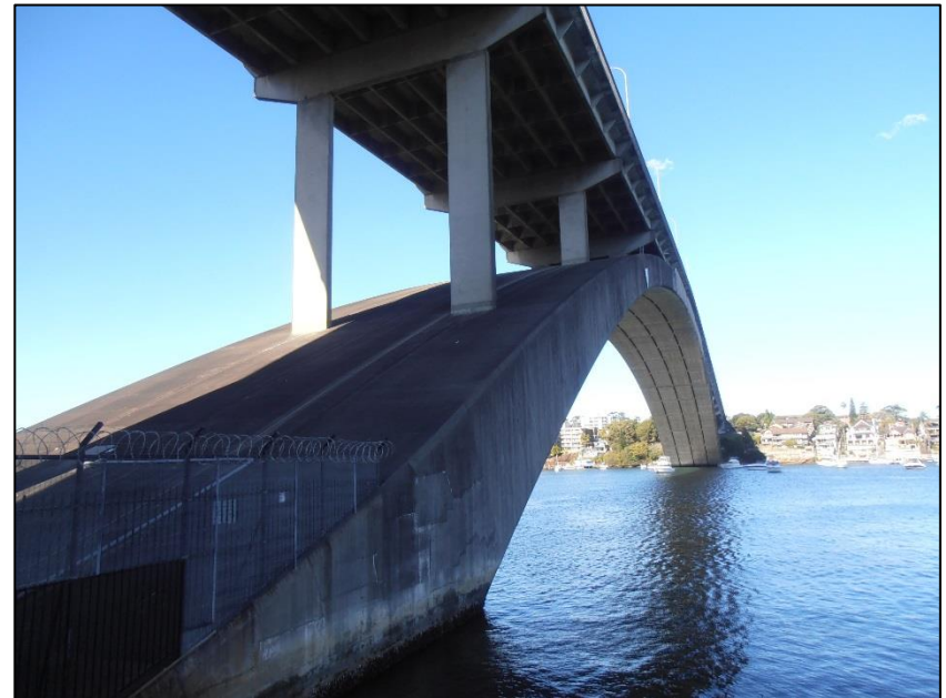
Gladesville Abutment (June 2014)
