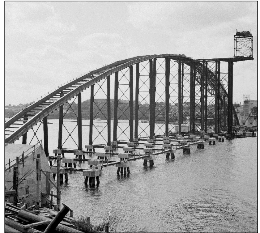
Note hoisting gantry for precast arch units
