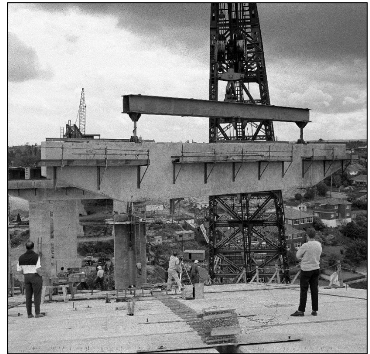
Precast concrete arch pier crosshead installation
