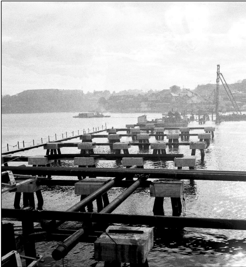
Note hoisting gantry for precast arch units
