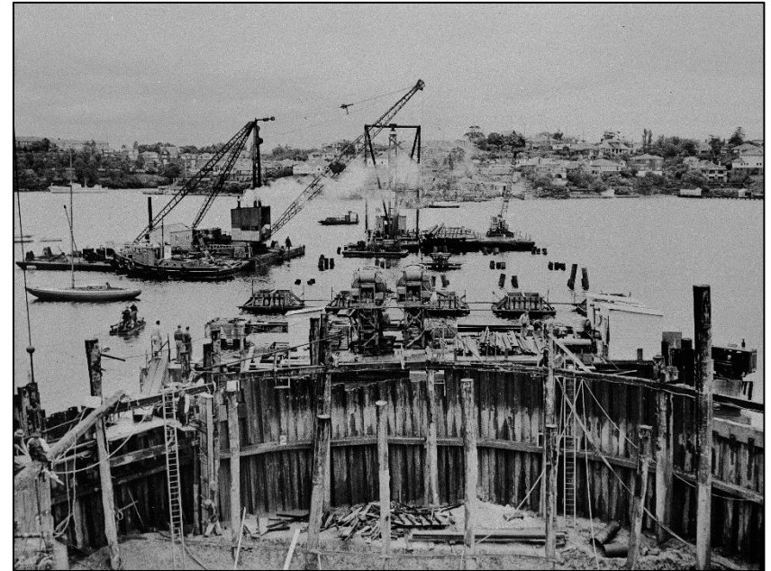
Timber sheet coffer dam under construction – Drummoyne side (1960)
