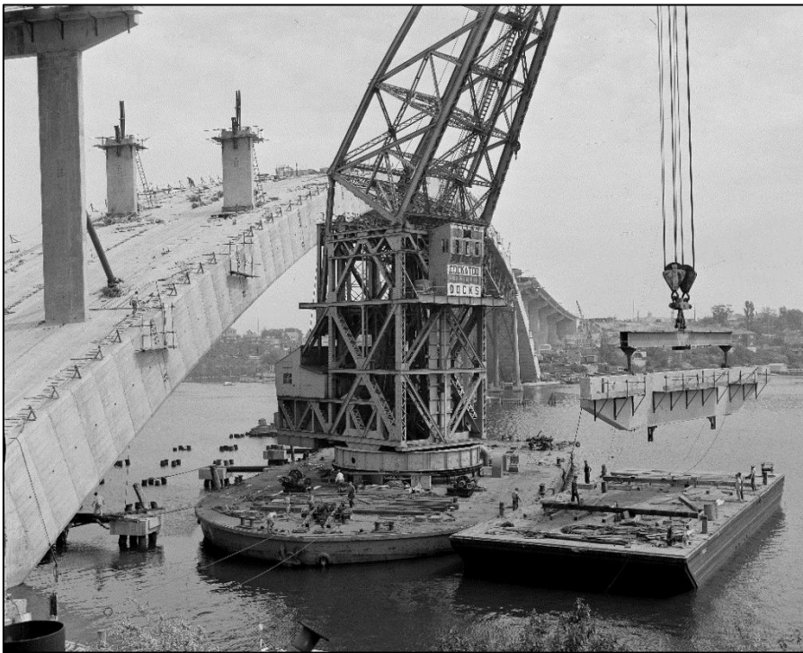
Precast concrete arch pier crosshead installation
