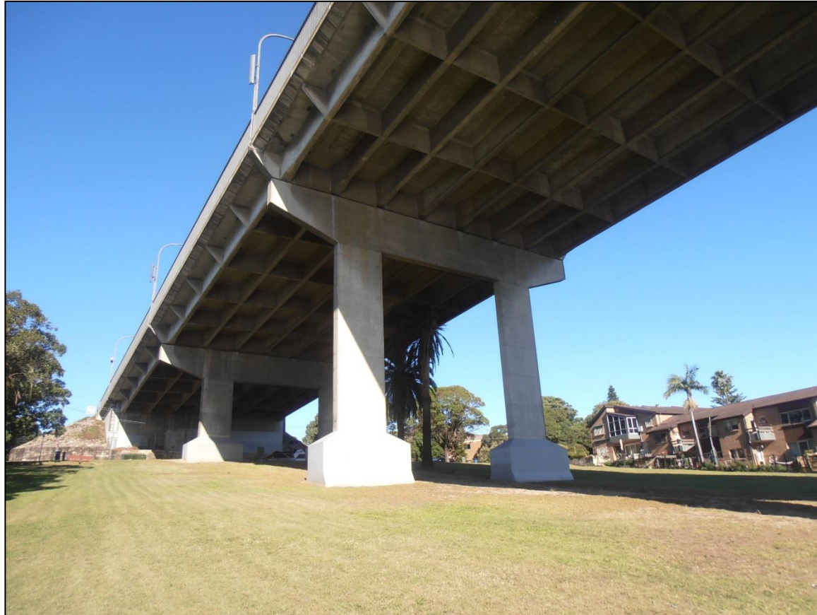
Insitu concrete used to complete beam and slab grillage
