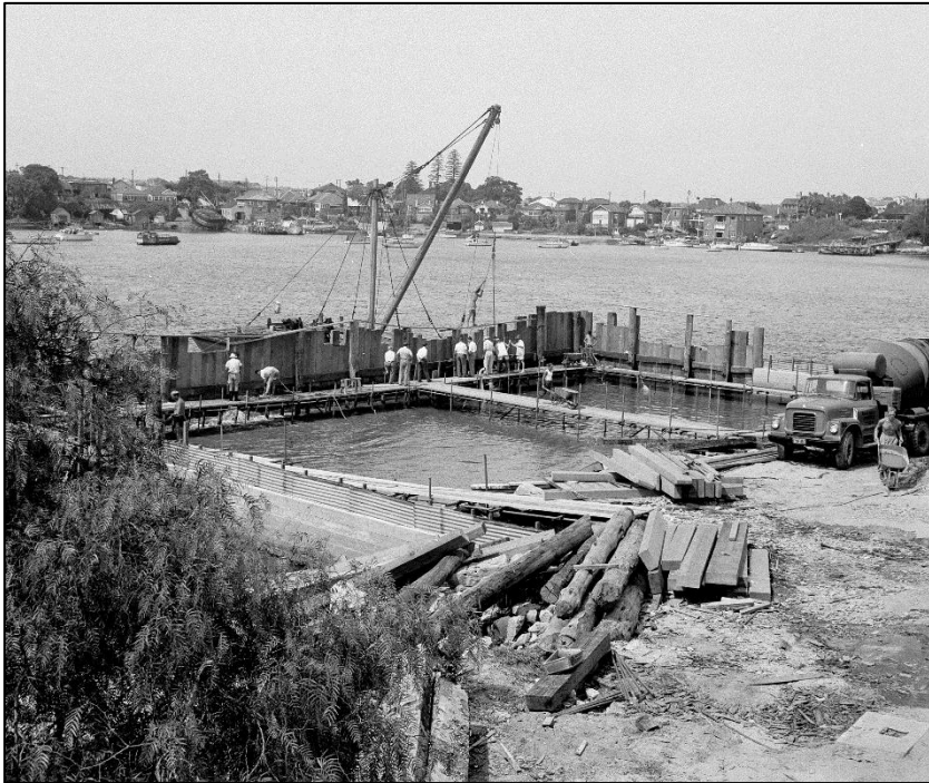
Timber sheet coffer dam under construction – Huntleys Point / Gladesville side (February 1960)
