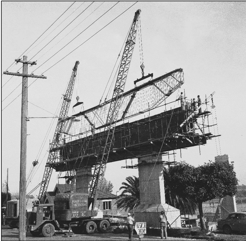
Cast insitu approach span piers
