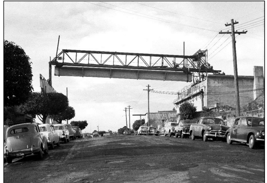
Launching gantry – approach span beams
