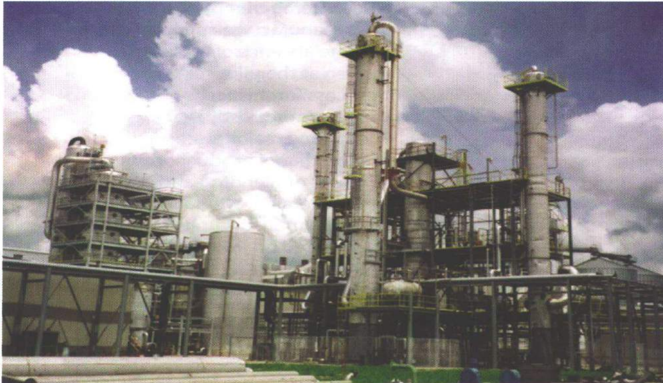
Ethanol from starch conversion plant
