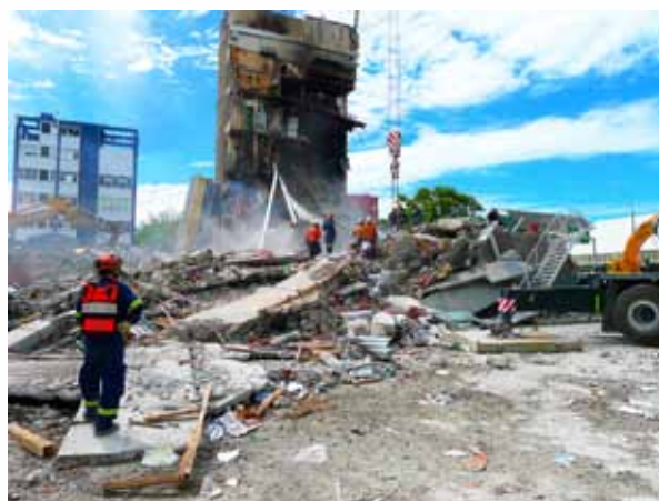
CTV building - only the lift tower was left standing
